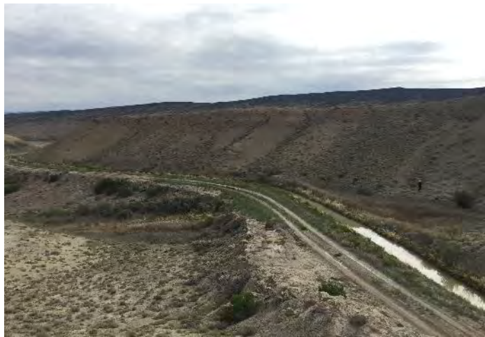
Photograph 1. Looking northeast along the EO Lateral in the North Project Area.
