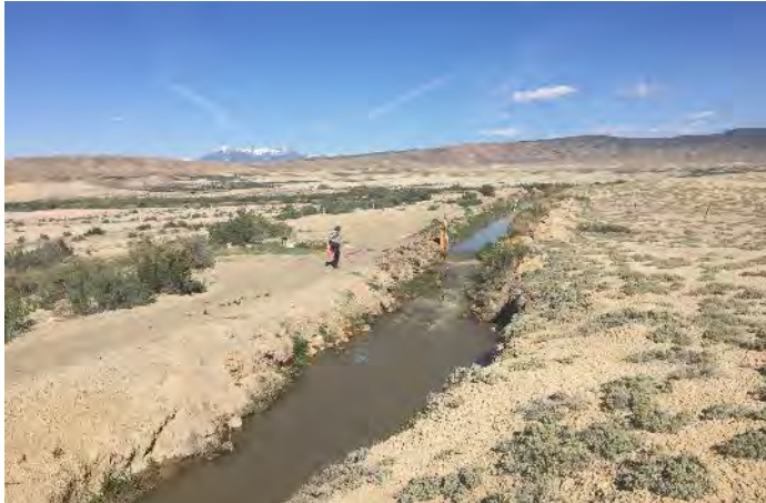
Photograph 2. Looking southwest along the GK Lateral in the North Project Area.
