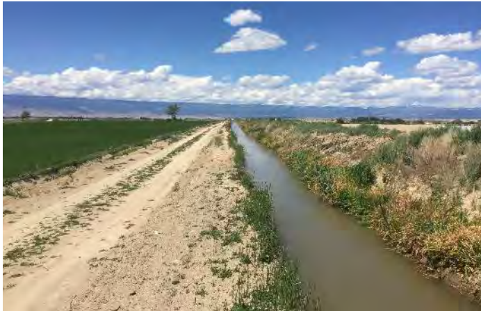
Photograph 5. Looking north along the GB Lateral in the South Project Area.
