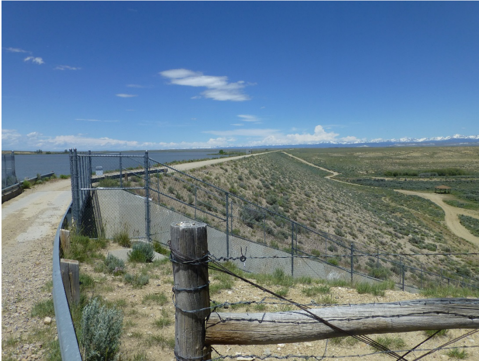
Figure D-1. Downstream face of Big Sandy Dam.
