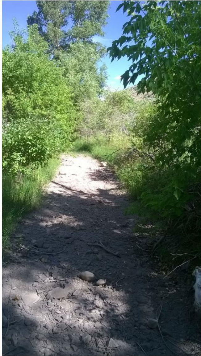
Photo 4: Typical Canal Cross-Section
