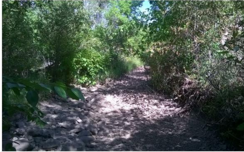
Photo 1: Typical Canal Cross-Section
