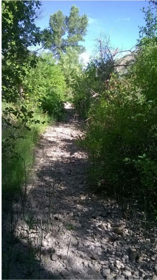
Photo 3: Typical Canal Cross-Section
