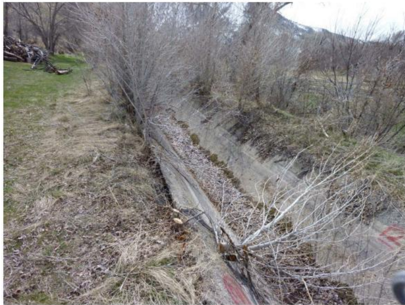
Photo 2: Typical Canal Cross-Section
