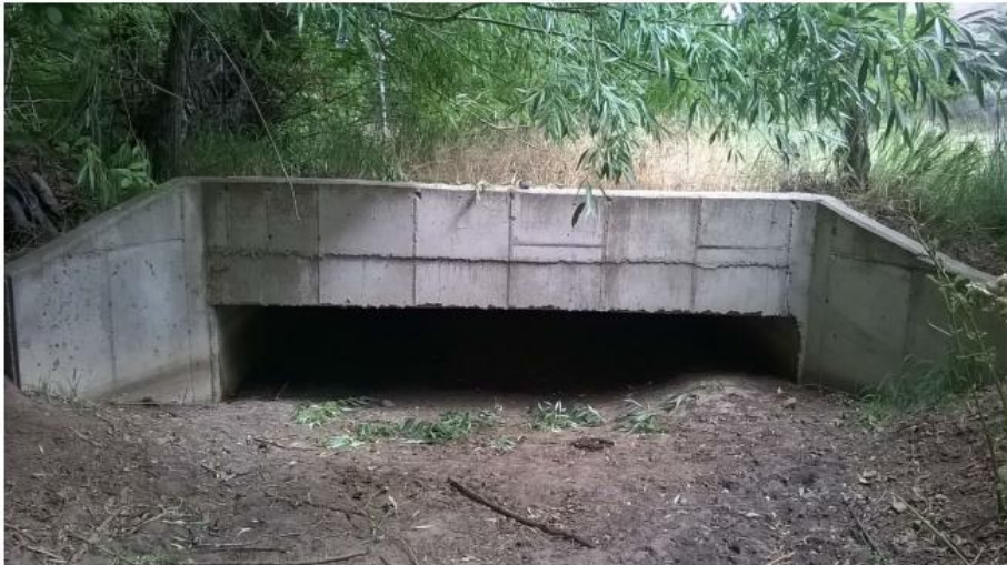
Photo 8: Box Culvert under Highway 40
