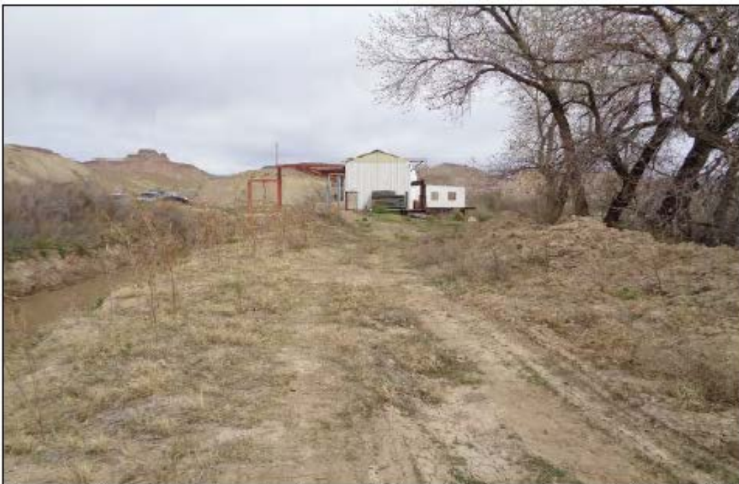
Photo 4. Thayn hydropower plant located at the end of the power canal, view north (north of Action Area #2)
