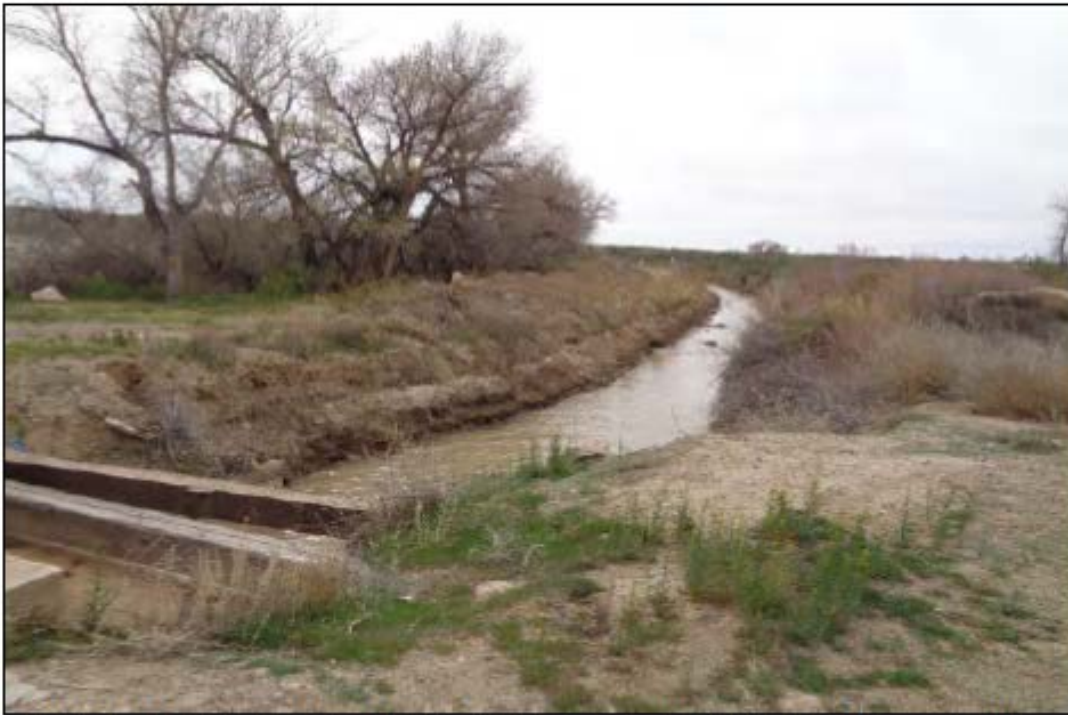
Photo 5. View southeast of Green River canal south of Thayn hydropower plant, looking towards center of Action Area #2
