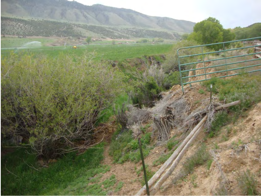
Photo 16. Segment N12, looking west.
