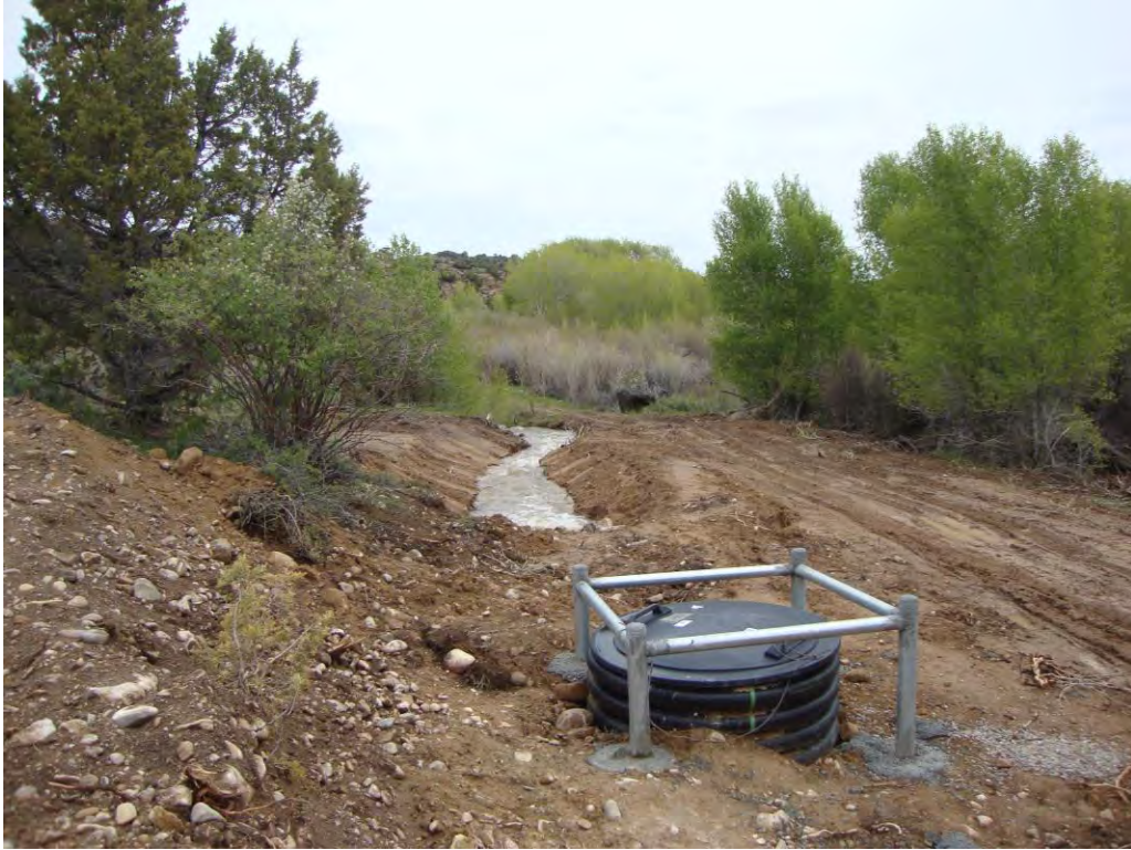
Photo 12. Segment N1 near diversion structure, looking northeast.
