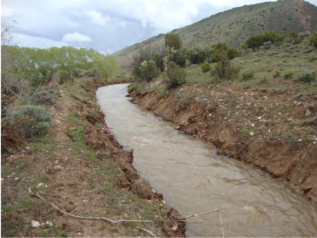
Photo 4. Segments A2 (in the background) and A3, looking south.
