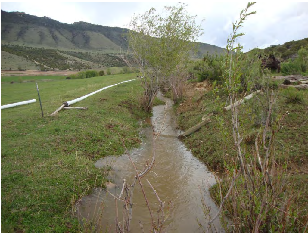
Photo 8. Typical section of the North Lateral through the farming area, looking southwest.
