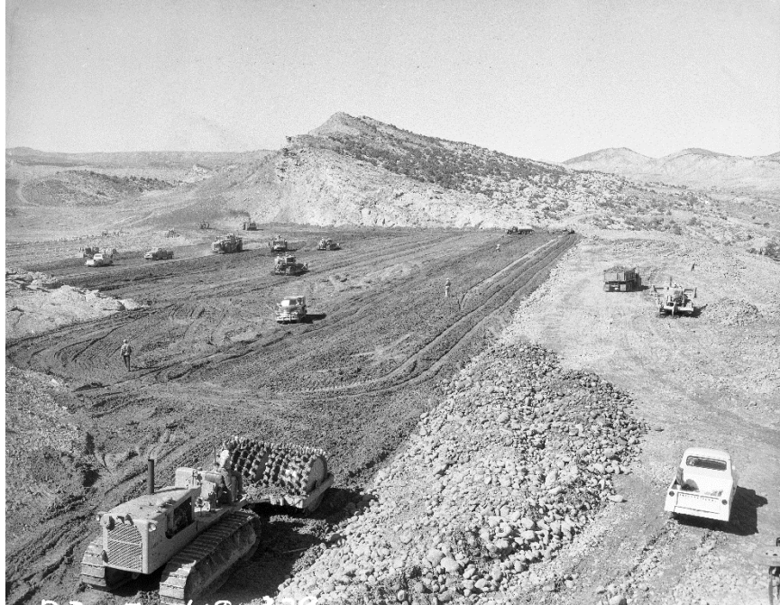
Figure 0.5 Embankment construction in progress on Zones 1, 2, and 3. View is looking northeast from right abutment. Average elevation for the three zones shown is 5450. Project photograph P325-418-0329, photograph by Elmer S. Davis, 7/18/1960.
