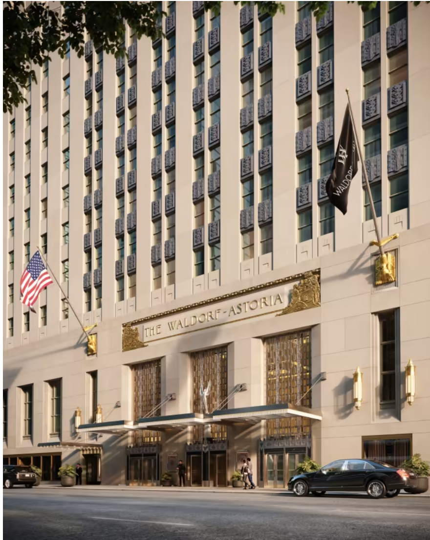
The Park Avenue entrance to The Towers at the Waldorf Astoria in New York © Noë & Associates/The Boundary
