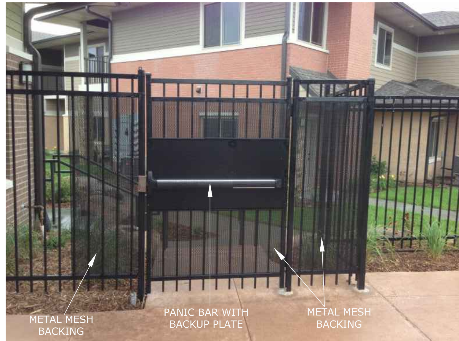
PEDESTRIAN GATE ILLUSTRATION USING A PANIC BAR WITH METAL MESH BACKING NTS
