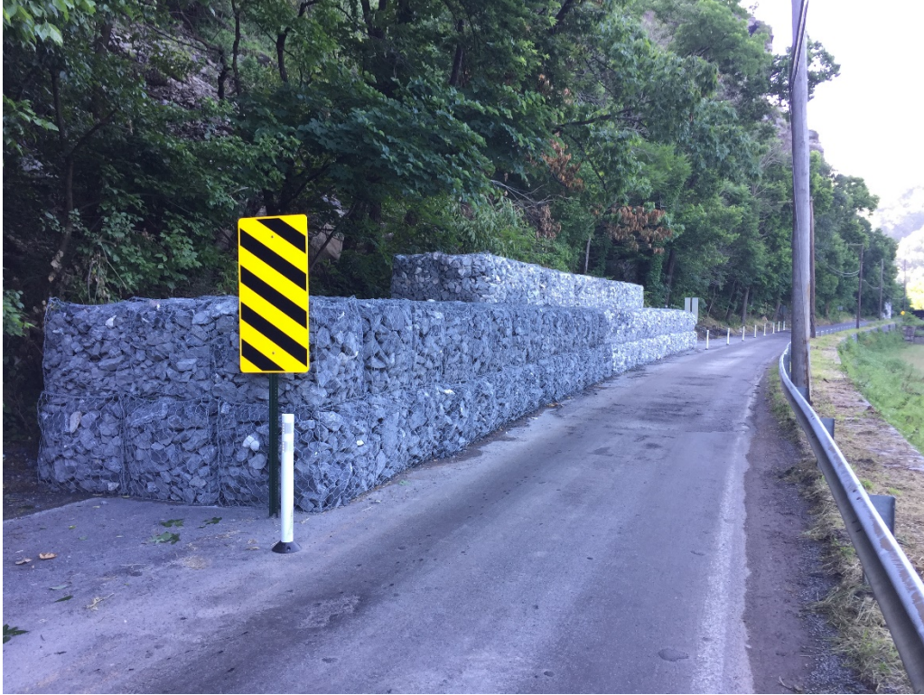
Photo 1: Sandy Hook Road Gabion Wall
