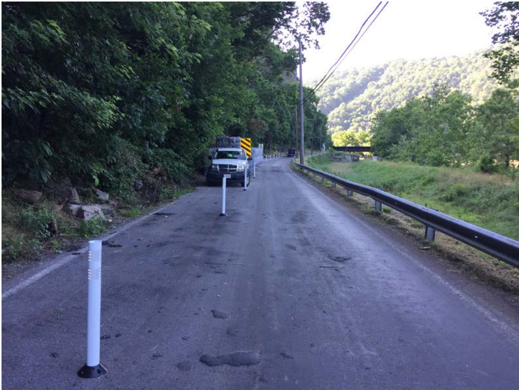
Photo 2: Sandy Hook Road looking East
