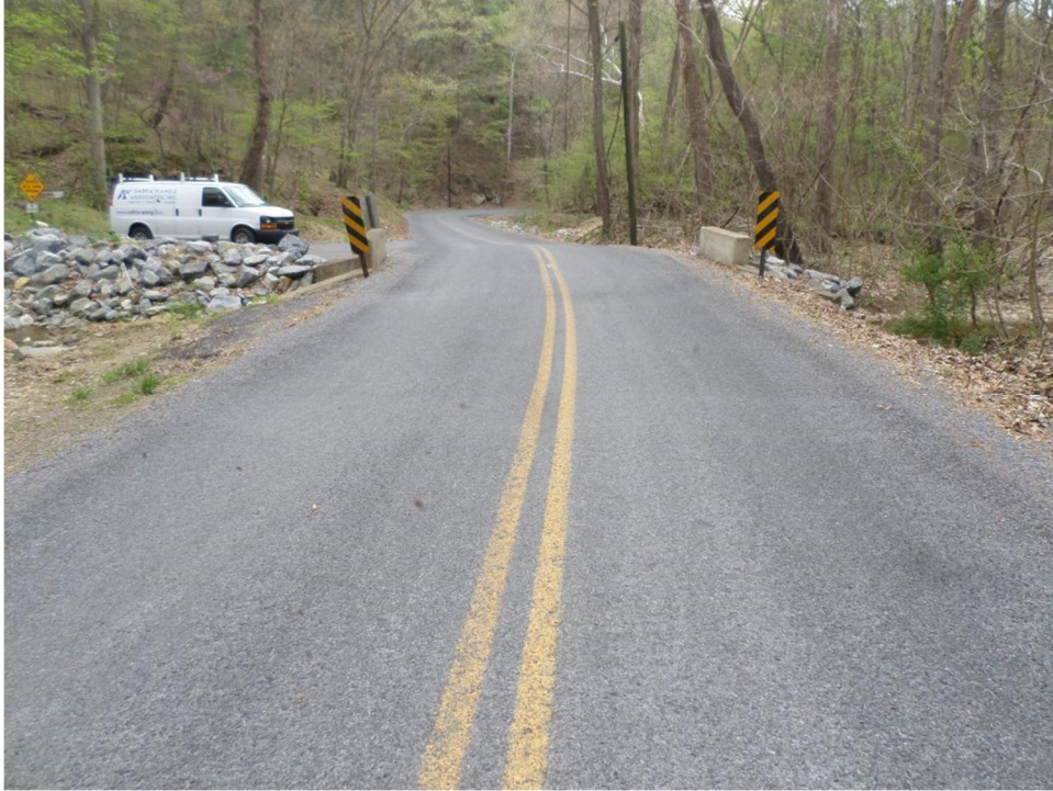
1. North Approach Looking South
