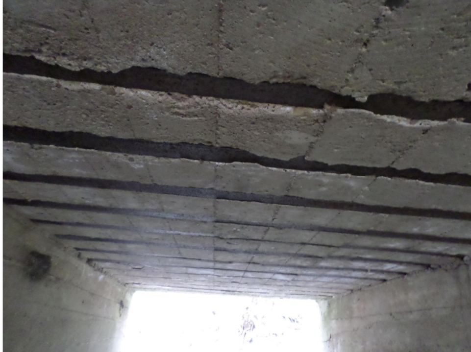
6. Exposed Bottom Flanges of Embedded Steel Beams at Original Bridge Slab
