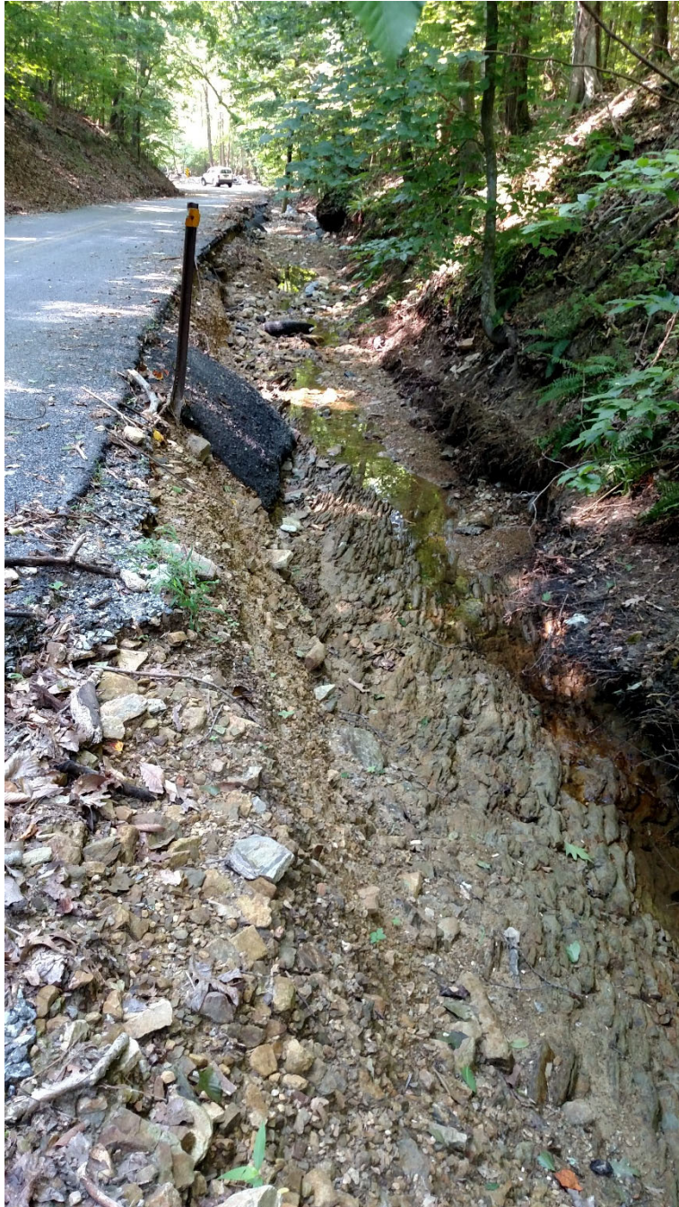
Back Road – Shoulder Repairs
