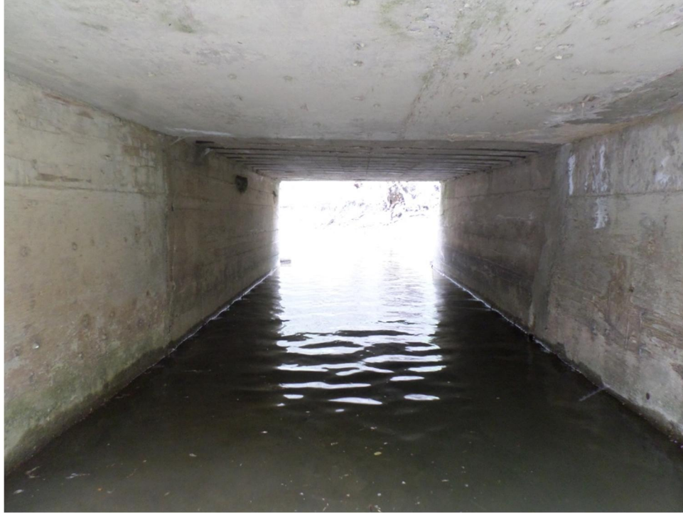
5. Typical Underside of Structure Looking West
