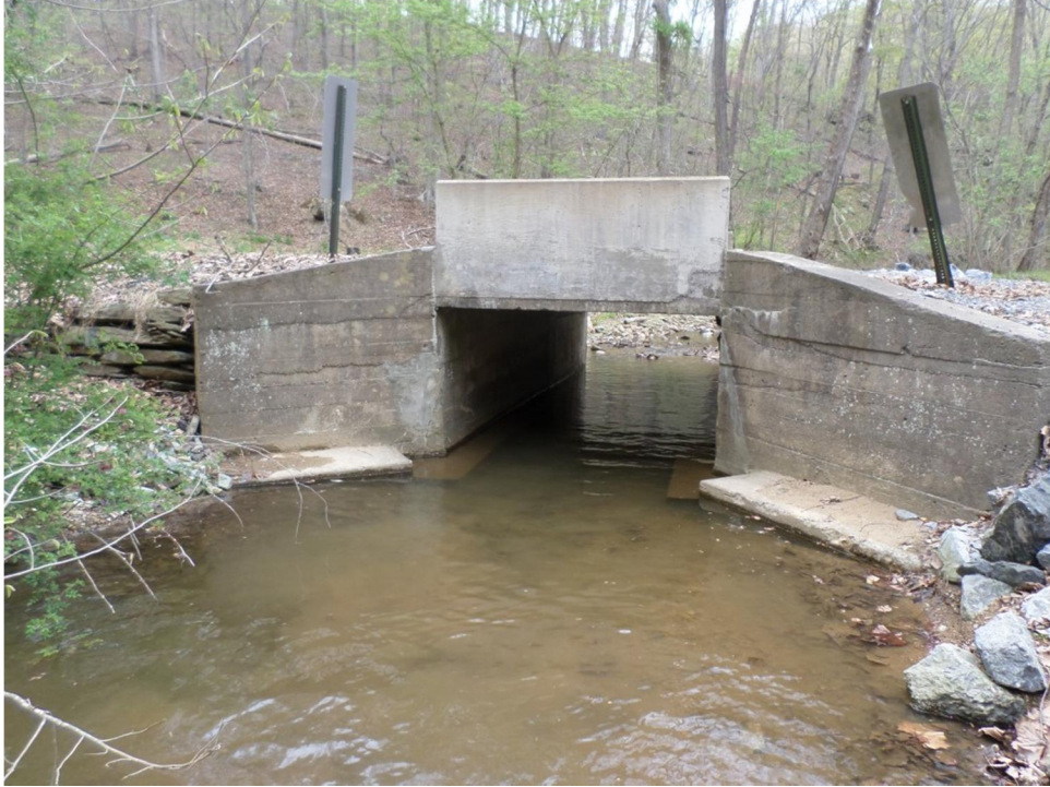
4. West Elevation (Downstream)
