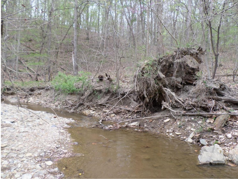
7. Moderate Erosion along Northwest Embankment (Note: Fallen Tree)
