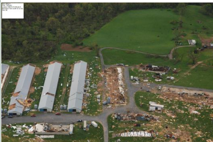
Shenandoah County Damage to a Poultry House
