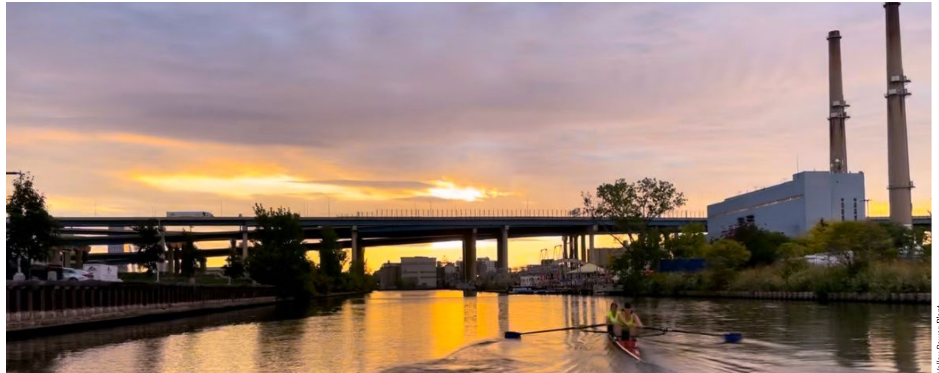
Valley Power Plant
