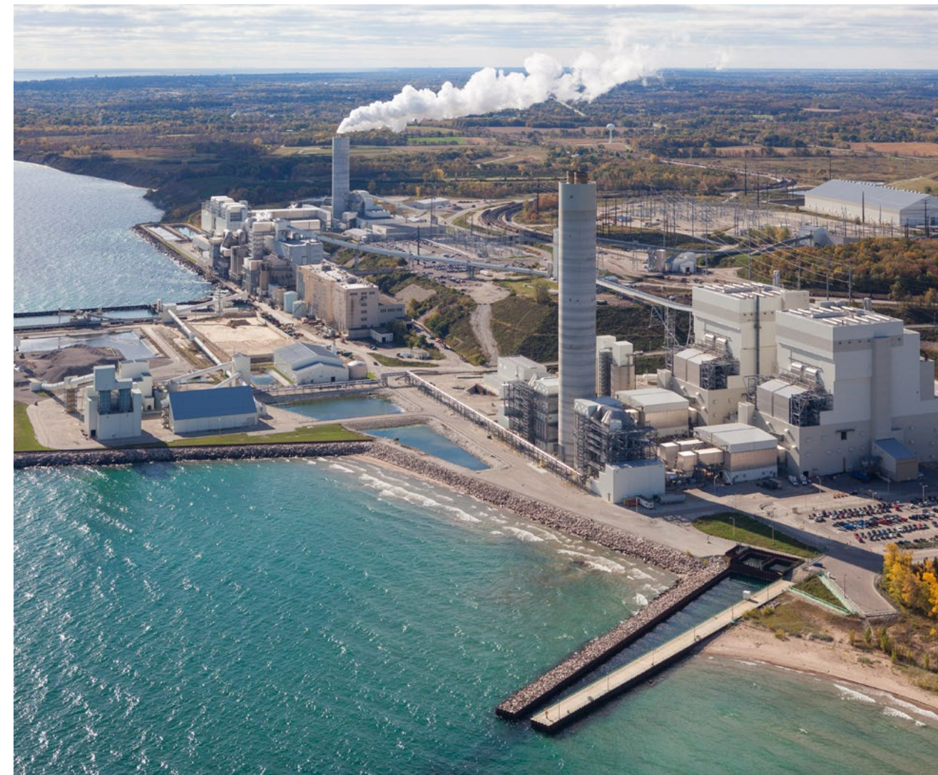
Oak Creek Power Plant
