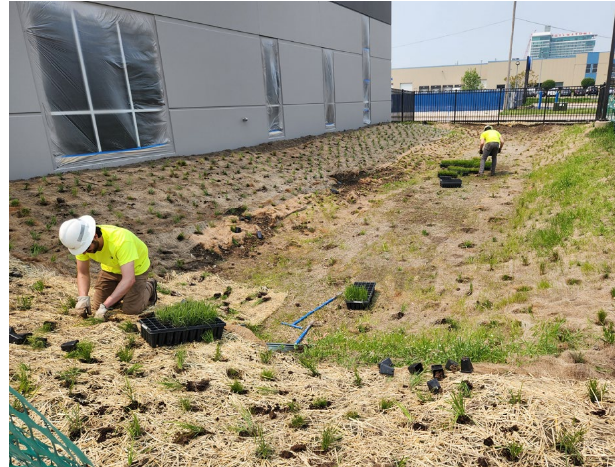
Installing native plants at the new District Energy Center in Milwaukee
