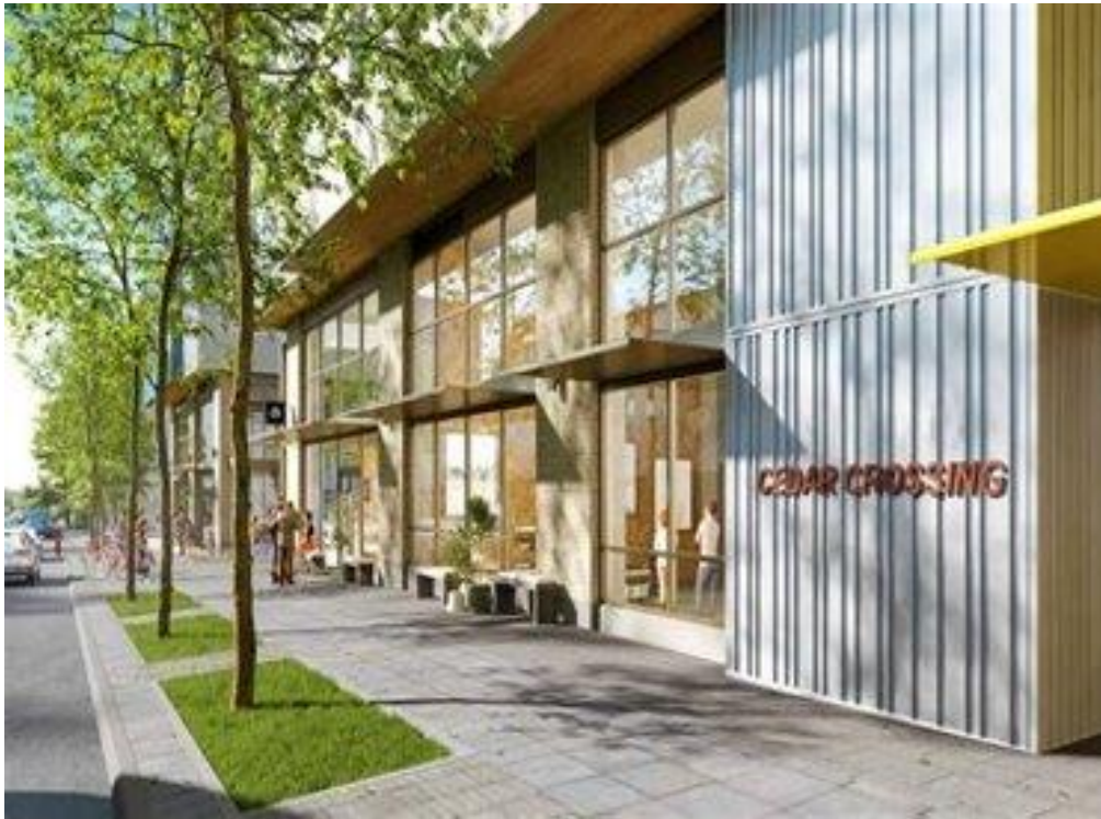
Photo courtesy of Bellwether Housing
