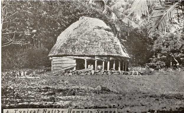
Figure 2. An early 20th-century photograph of a fale, a thatched pavilion without walls.
