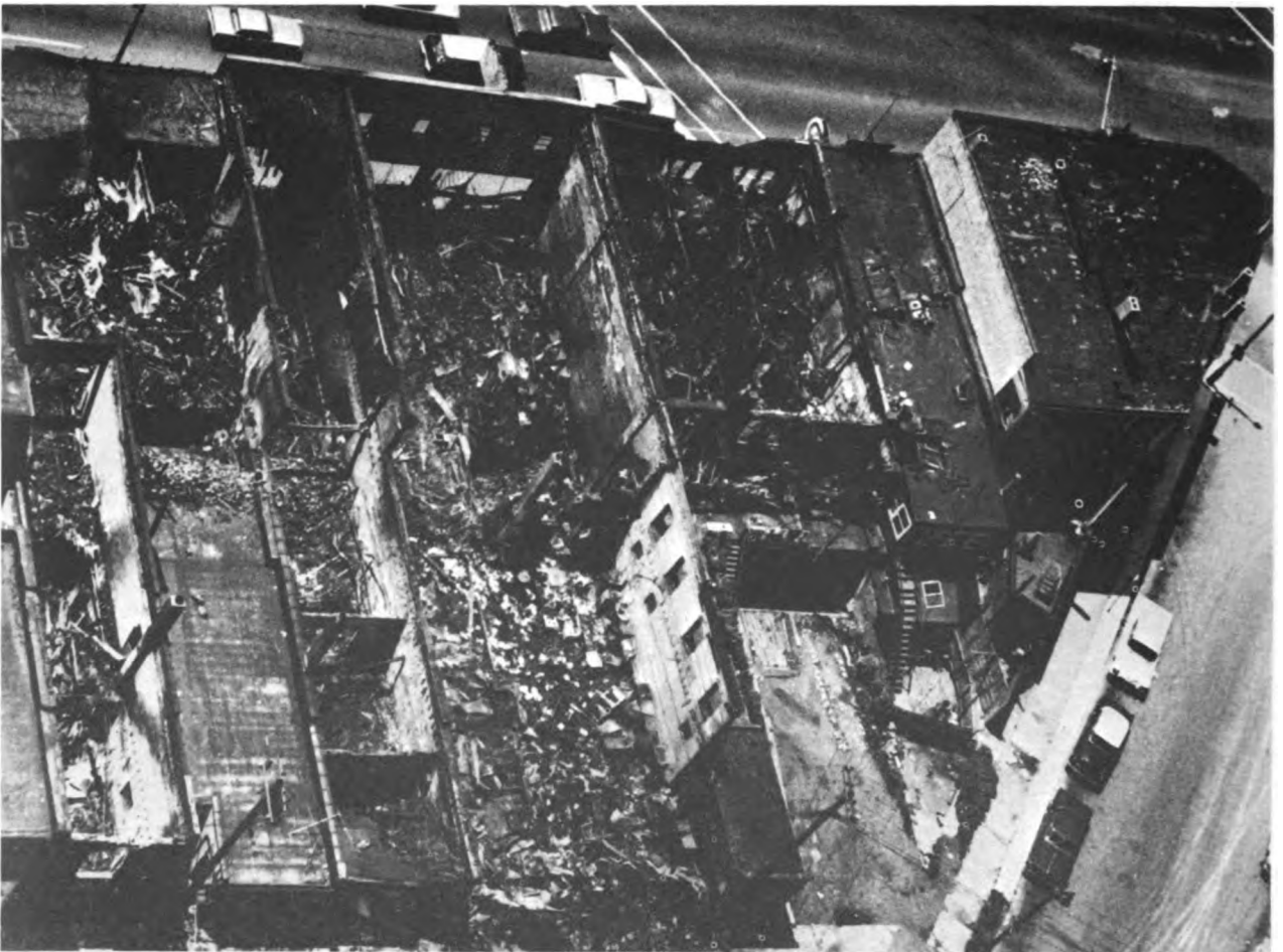
Gutted buildings, Detroit
