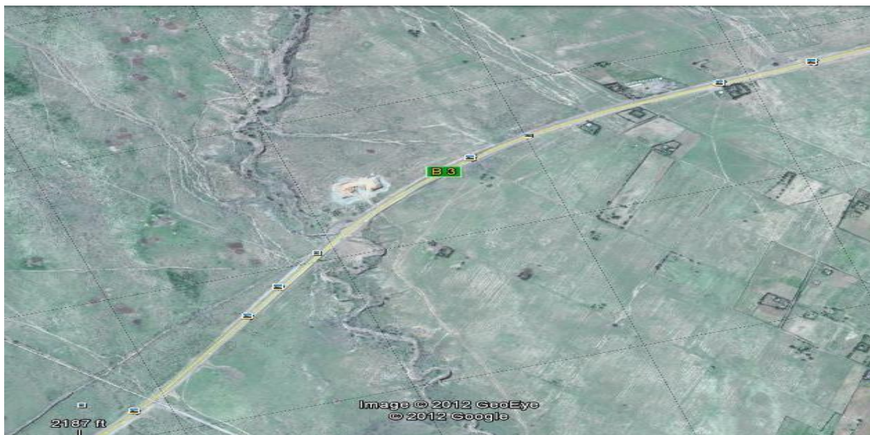
Figure 47: Section of the road that was washed away
