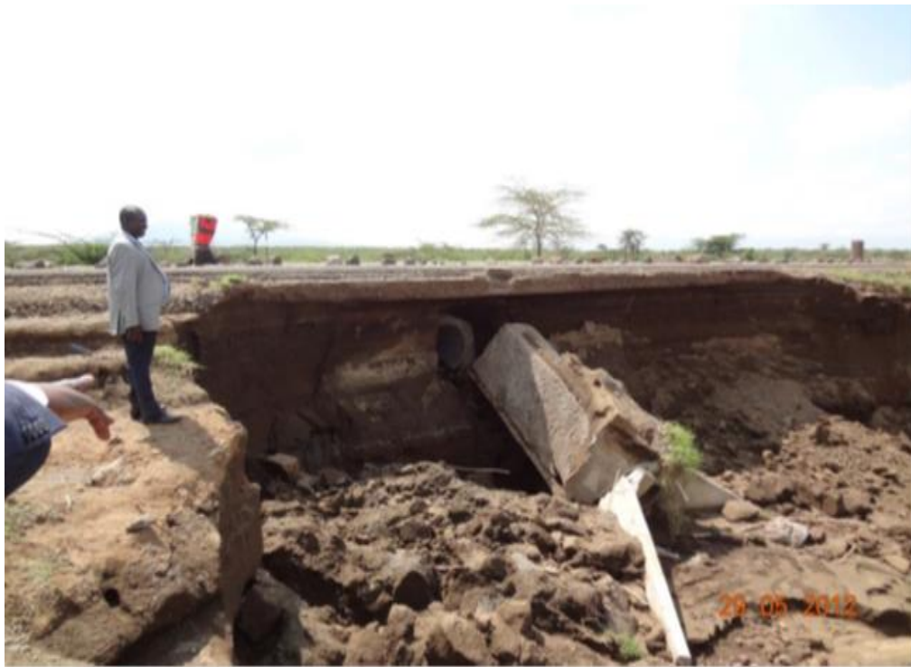
Figure 62: Road surface remained intact.
