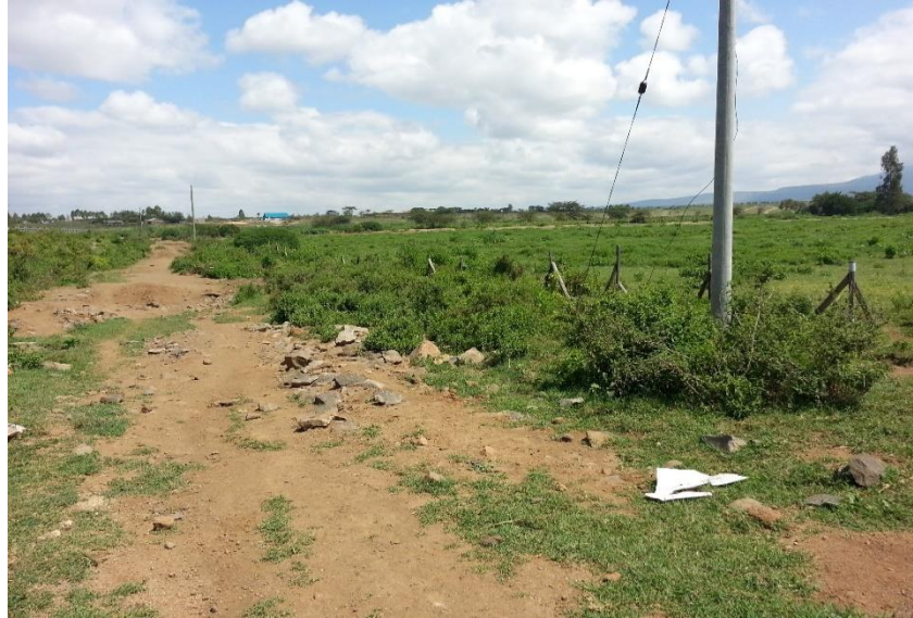
Figure 5: RHS of the fissure on Maai Mahiu road
