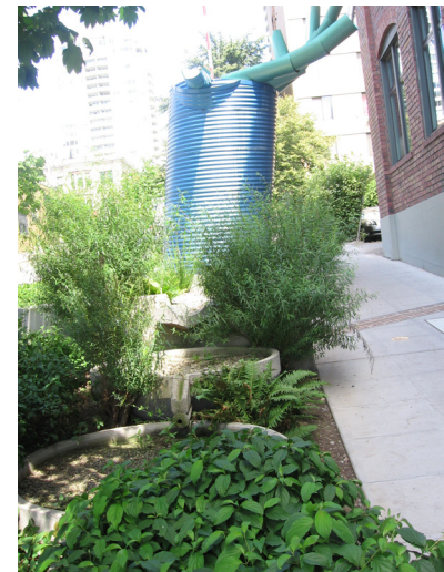
Vegetation and creative rainwater catchment features can add interest to a streetscape and help to address stormwater run-off.
