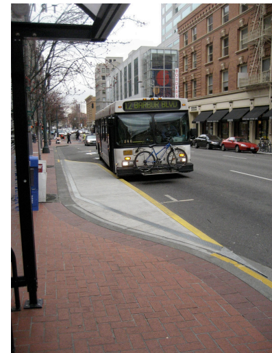
Curb extensions and transit shelters define transit stops and provide safe and comfortable conditions for riders.
