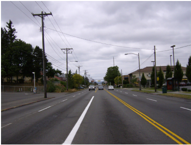
The Avenue Complete Street typology emphasizes "road diets", or reducing the typical 5-lane cross-section to 3 or 4 lanes where functionally feasible.
