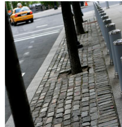
Pervious pavement treatments may be appropriate where there is limited room in the sidewalk/amenity zone for providing optimally sized tree pits. Tree grates may also be used if it is necessary for tree pits to encroach into the sidewalk zone.
