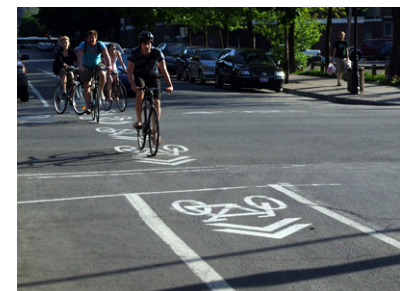
Where there is adequate room, bicycle facilities (lanes or sharrows) should be continued through the intersection.
