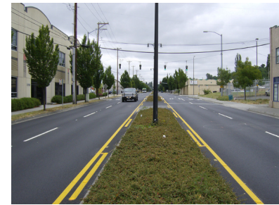
This median in the Lower Portland Mixed-use Center restricts turn movements, reduces vehicle conflicts, and visually enhances the roadway.
