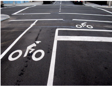
Bike boxes improve visibility and safety of bicyclists at intersections by clearly defining the bicycle and vehicle zones and allowing bicyclists to get a head start across the intersection.
