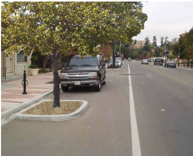
Tree bulbs may be placed in the parking zone where there is not enough room in the amenity zone.
