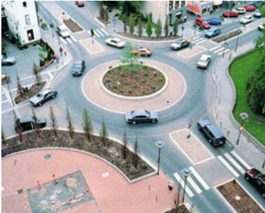
Roundabouts may be considered for intersections, and may serve as gateway features for Mixed-use Centers.
