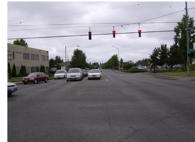
Pedestrian Streets within Community Centers such as Tacoma Central typically are 5-lane arterial streets. The Avenue Complete Street typology may be applicable to such roadways.
