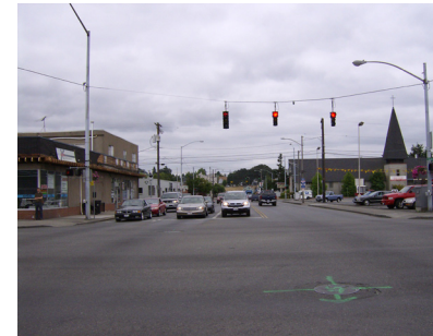
S. 56th St. within the 56th and South Tacoma Way Mixed-use Center.
