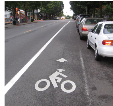
Bicycle lane marking.
