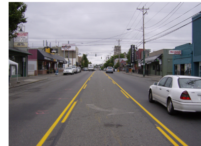
Pedestrian Streets within Neighborhood Centers such as 6th and Pine typically are 3-lane arterial streets with on-street parking. The Mainstreet or Transit Priority Complete Street Typologies may be applicable to such roadways.
