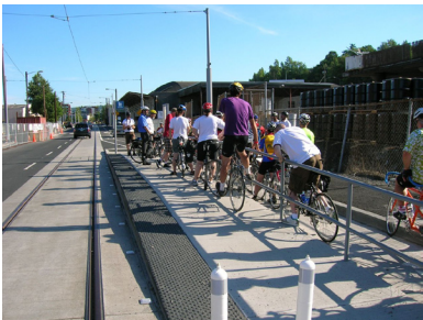
The City of Portland has designed a grade-separated bicycle lane that circumvents streetcar stops in order to address conflicts that result from curb extension platforms where there are bicycle facilities.
