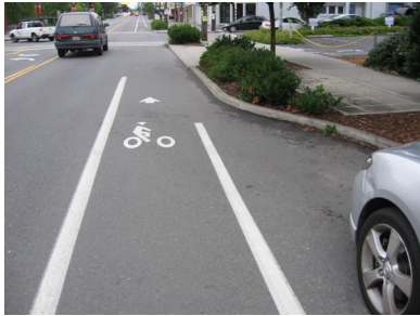
The parking lane should be defined by a solid painted line to ensure an orderly alignment of cars when adjacent to a bicycle facility.
