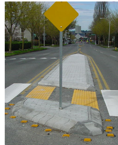
Median with mountable curb and pedestrian refuge.
