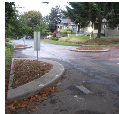
Chicanes and traffic circles are traffic-calming elements that can be used along bicycle boulevards.
