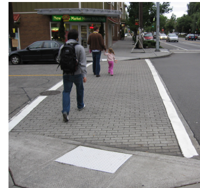
Special pavement treatments such as stamped concrete help to clearly define the crosswalk and add visual interest.
