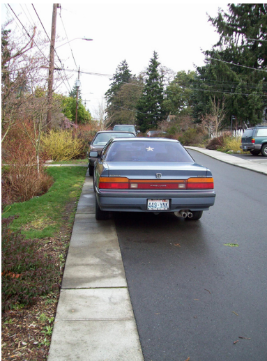
Flattened curbs allow for sheet flow of stormwater into roadside natural drainage facilities while providing an edge to the roadway.
