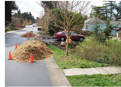
Natural drainage systems require periodic maintenance, including mulching, replacement of bottom soil, and pruning of vegetation.
