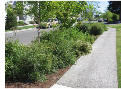
Sidewalk constructed of pervious concrete.
