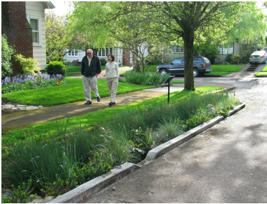
Curb extension with rain garden.
