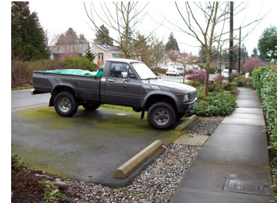
In certain situations where the objective is to reduce roadway width to the fullest extent possible to meet stormwater management goals, parking may be provided in clusters adjacent to the roadway.
