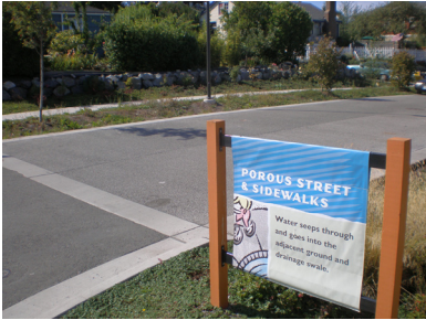
Stormwater flows may be reduced by using permeable pavement for sidewalks, driveways, and in some cases, within the roadway.
