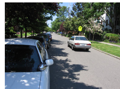
Skinnier roadway widths reduce impervious surface and associated stormwater flows.
