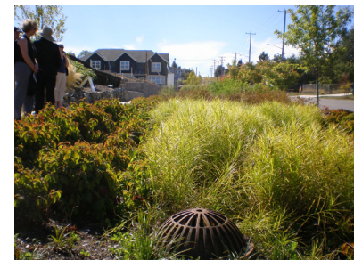
Appendix 3 of the Low Impact Development Technical Guidance Manual for Puget Sound contains specific guidance plant species that are appropriate for natural drainage features.
