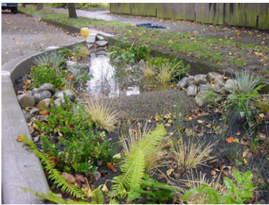
Rain garden within a curb extension.
