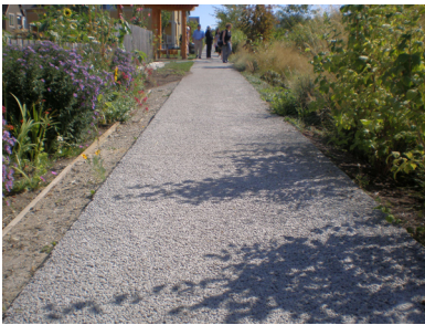
Sidewalk constructed of pervious concrete.
