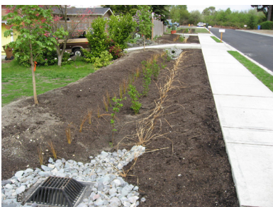
A bioretention swale built along Visscher St in Tacoma.
