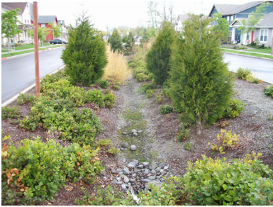
The Salishan housing development contains many low impact development features, including this rain garden within a street median.
