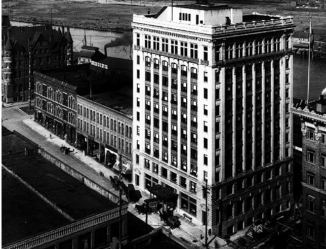
The 1912 Tacoma Building at 1021 A Street housed the headquarters of the Weyerhaeuser Company until the late 1960s. More recently, it was rehabilitated into a modern office building. (Source: University of Washington, Digital Collection)
