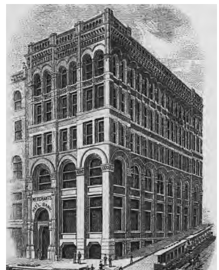
The 1891 Merchants National Bank building at 11th and Pacific was demolished in the early 1960s.
