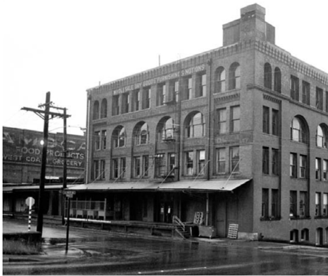
Historic resources provide visitors with a glimpse into Tacoma’s heritage while allowing for new economic development such as the rehabilitated Garretson Woodruff Pratt building on the University of Washington Tacoma campus. (Source: University of Washington, Digital Collection)
