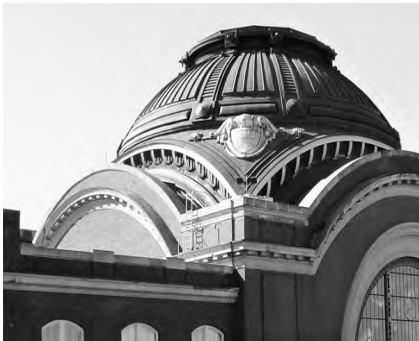
Union Depot's copper dome was replaced in 1994 after 83 years of service.
