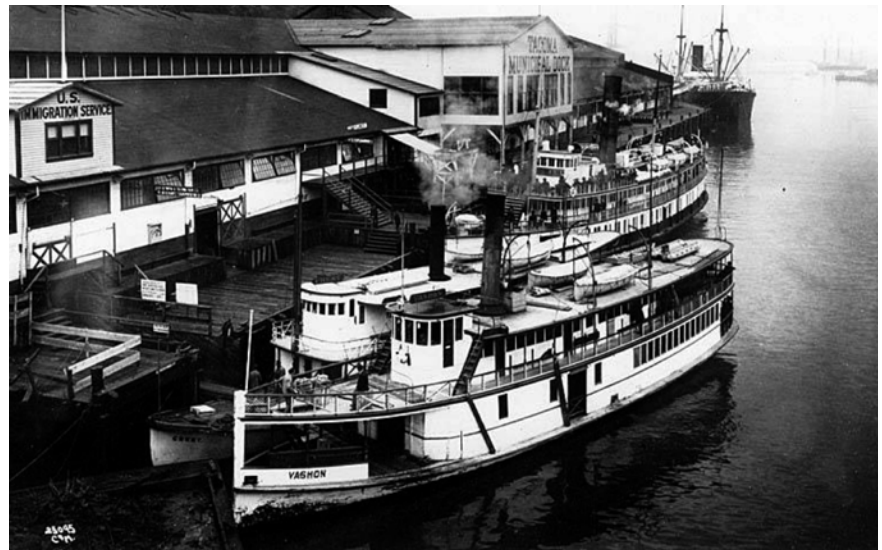
The steamers Flyer, Vashon and Crest docked at the 1911 Tacoma Municipal Dock which was demolished in the early 2000s. (Source: University of Washington, Digital Collection)
