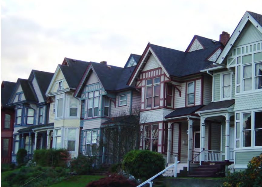
The South J Street Historic District consists of a row of intact Victorian Era homes.
