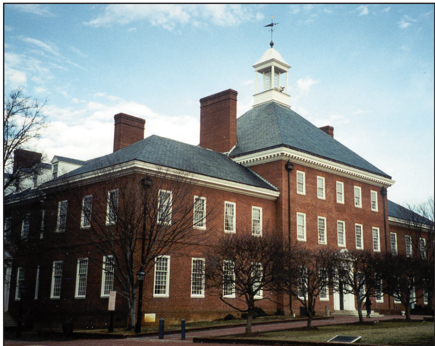
The Legislative Services Building houses staff to the Maryland General Assembly.
