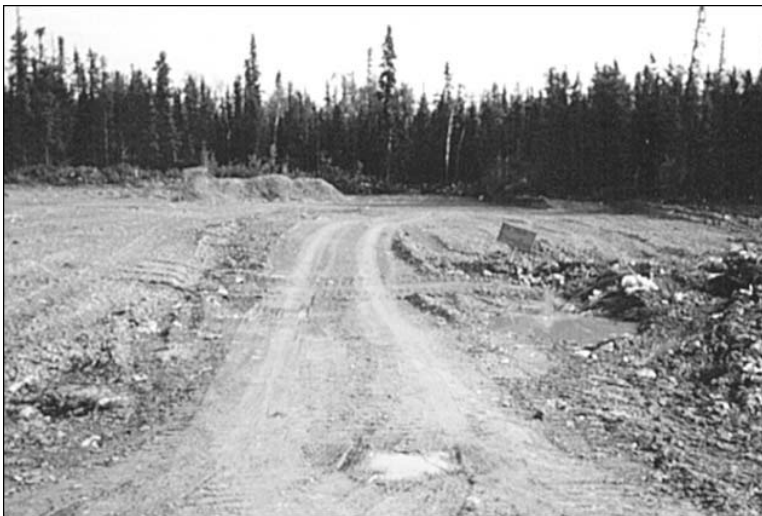
A landfill with covered wastes.
