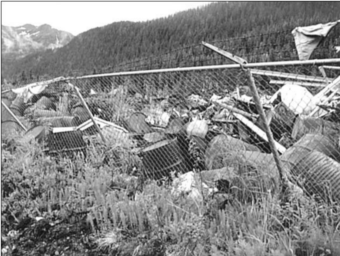
A fence in poor repair surrounding a landfill.
