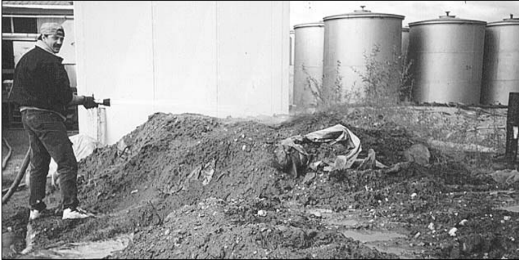
Treating contaminated soil.
