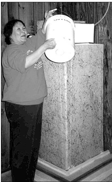
Honey bucket disposal system.
