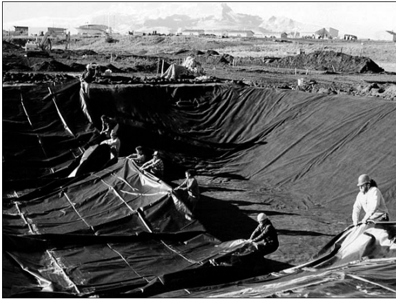
Building a sewage lagoon with a liner.
