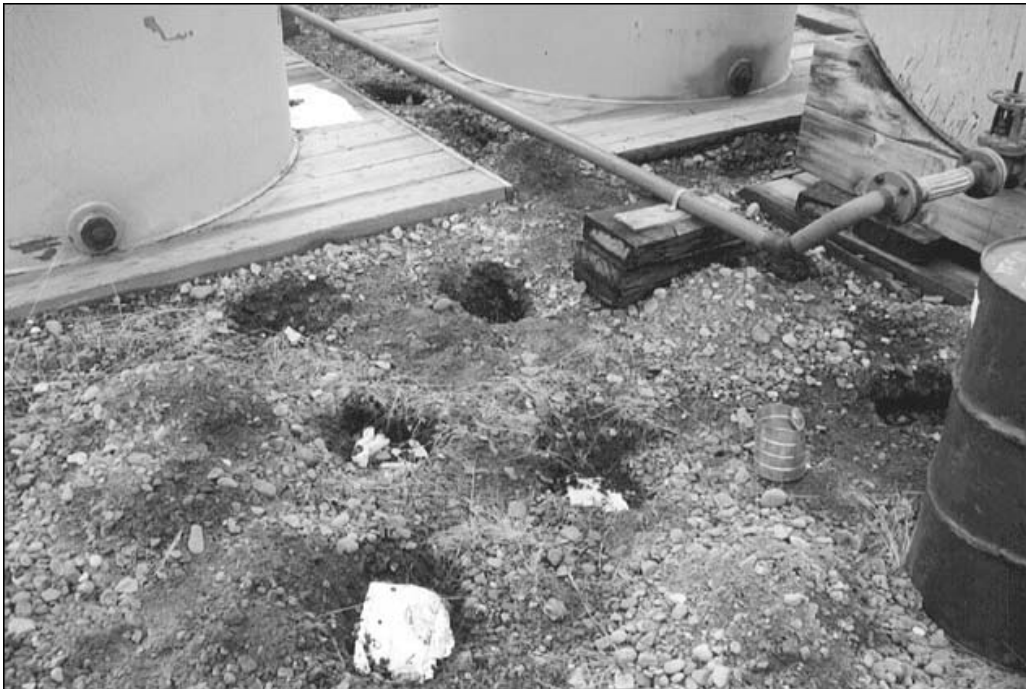
Active fuel spill at a tank farm.
