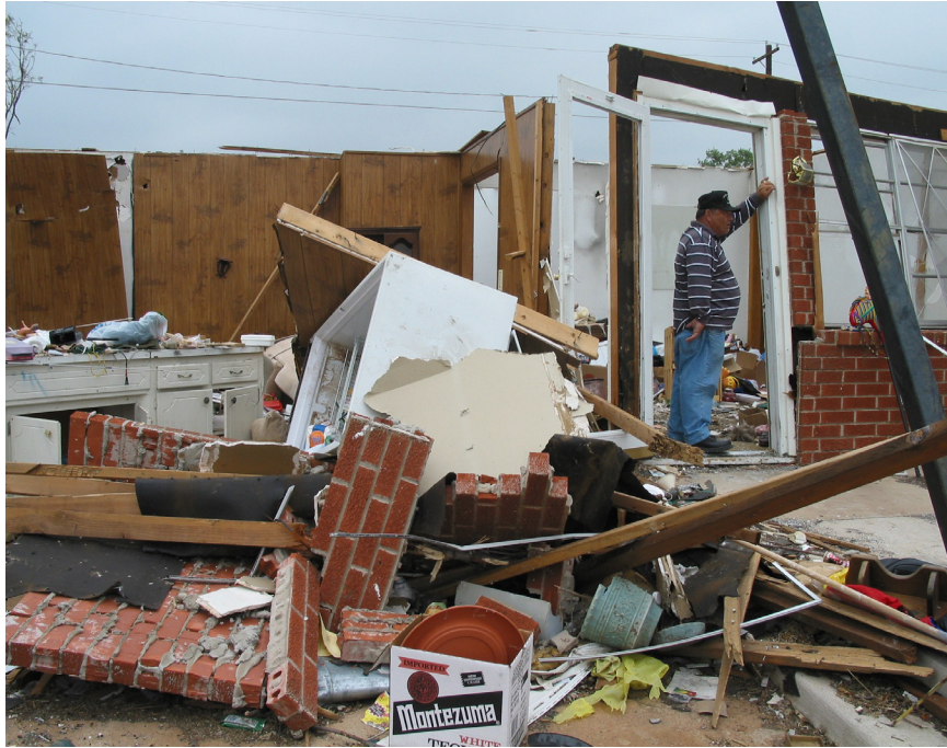
Figure 6. The May 8, 2003, tornado damaged or destroyed hundreds of buildings in Moore.
