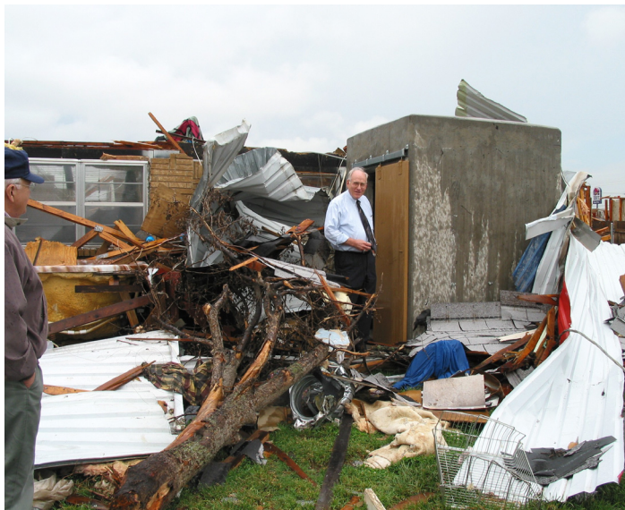
Figure 7. Dr. Ernst Kiesling, Texas Tech University researcher, inspects an above-ground SafeRoom that survived the 2003 tornado in Moore.
