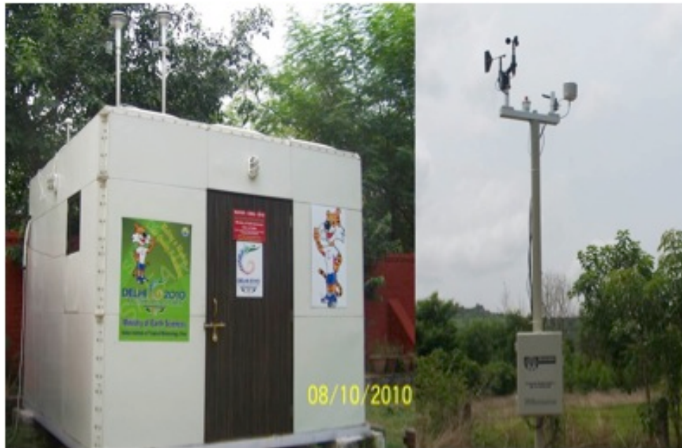
Figure 14c. A monitoring station located in NCT
