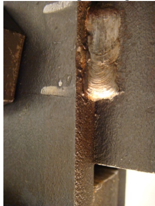
Figure C-29: Longitudinal weld fatigue crack in specimen TW-2TN-12-1
