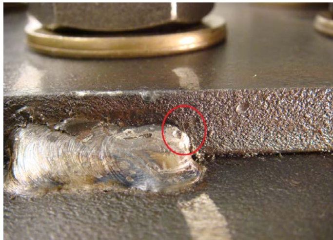
Figure C-10: Front face lower left tack weld toe crack for specimen TW-3LN-20-3
