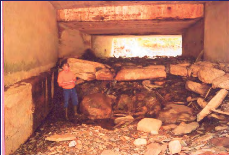
Rte. 36 / Rock Spring Creek 9/2003 --- Note: Spread Footings on earth
