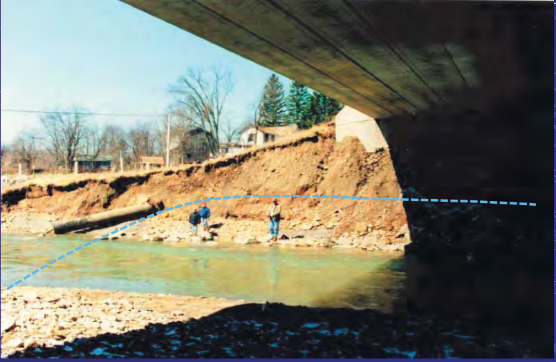
Install River Training Structures
