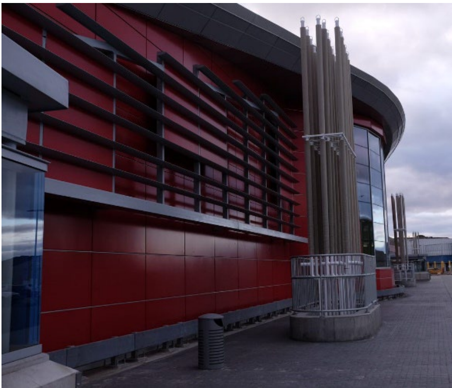
Iqaluit airport was built with a system of ‘thermosyphons’ to draw away heat before it reaches the permafrost below.
