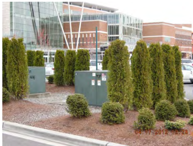
Figure 18-48: Using evergreen landscaping to screen utilities
