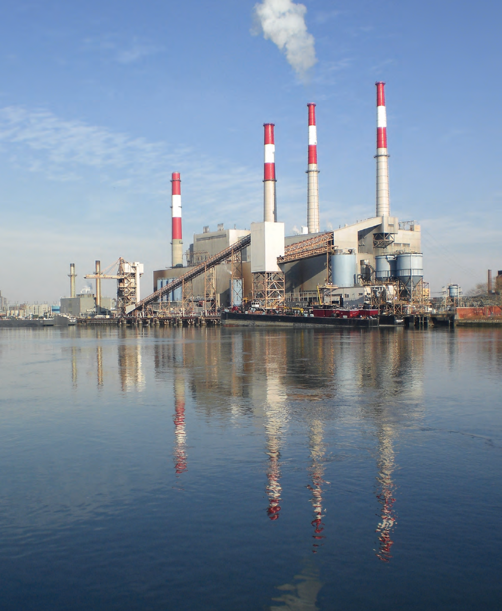
Ravenswood Generating Station, on the East River waterfront, is the largest power plant in New York City.
