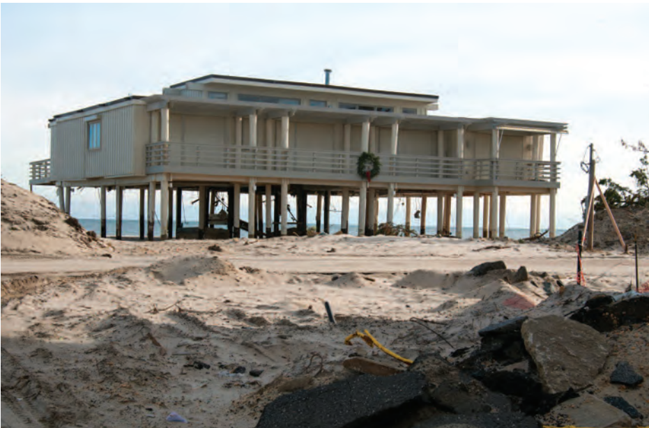
Residential home in New Jersey, compliant with FEMA standards
