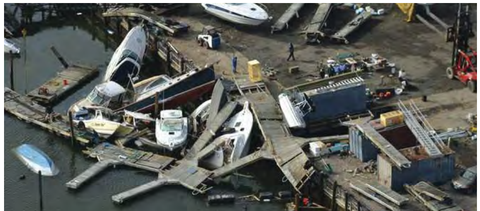
Damage at Great Kills Marina
