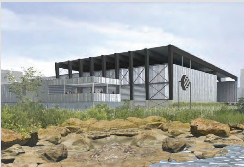
The future Sims Municipal Recycling Facility, located at the South Brooklyn Marine Terminal, will be elevated above the Base Flood Elevation
