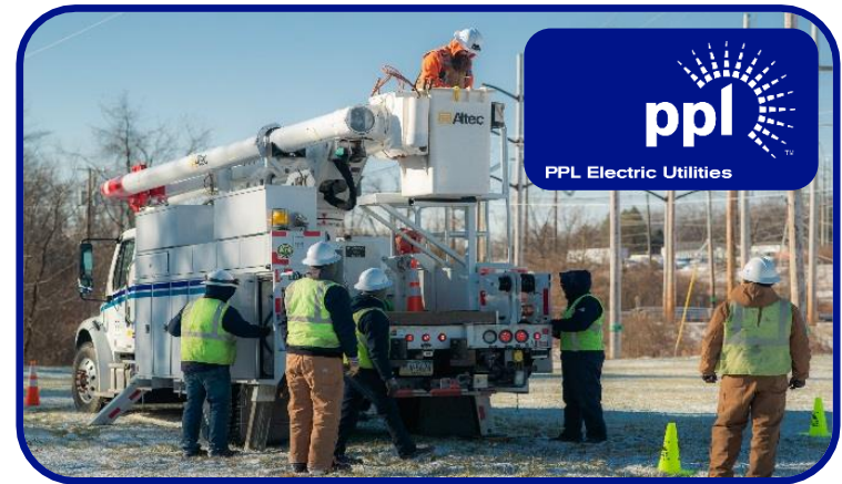
Employees testing new downed wire technology
