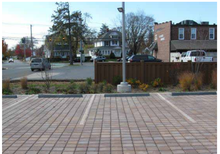
Permeable pavers are a river-friendly substitute to concrete and asphalt. Removing curbs and directed flow into rain gardens captures stormwater. Source: US EPA
