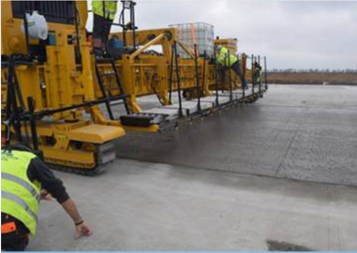
SPRAY BAR MOUNTED ON T/C MACHINE
