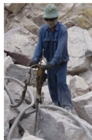
Figure 3 Picture of Tool Operator
