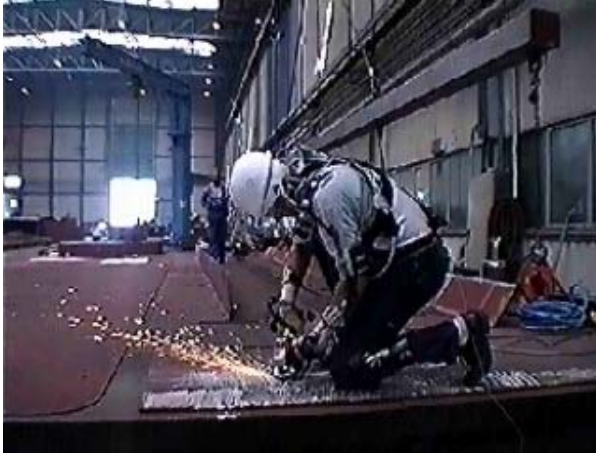
Figure 1 Preparation of the weld seam with an angle grinder
