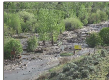
Colockum Creek Road Washout, WSU Chelan-Douglas Extension
