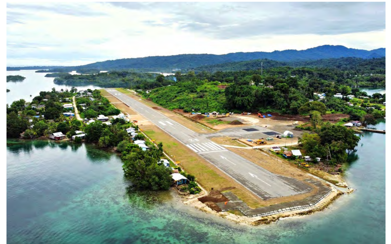
Photo by Downer Group
