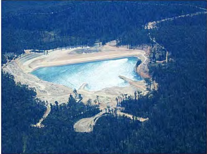
Plate 1. Aerial view of the Benambra tailings dam at completion of rehabilitation works.
