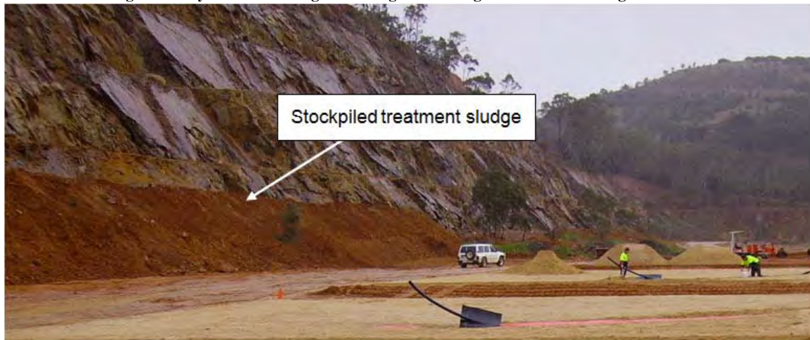
Figure 1: Dry treatment sludge stored against the highwall at the Brukunga mine site.
