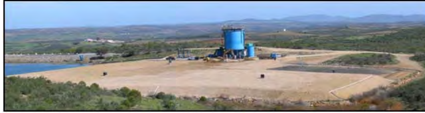
Figure 5-14: Test Plot for Paste Tailings - Somincor Neves Corvo Mine, Portugal
