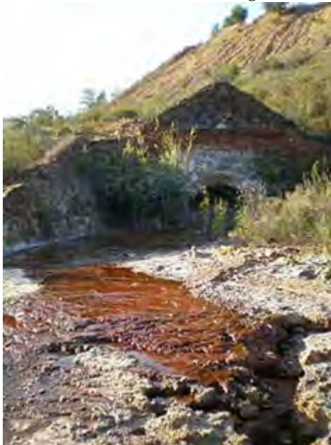
Figure 2: Roman Portal with Acid Rock Drainage – Spain
