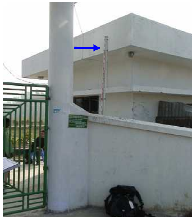
Fig. 4.8 Water mark on the wall of botanical garden
