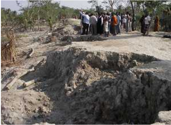
Fig. 1-3-5 Outer sea banks damaged by the storm surge
