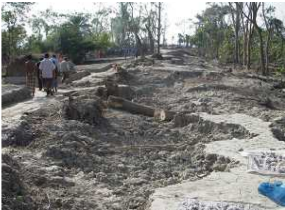
Fig. 1-3-6 Bank Slope being tampered for encroachment by landless people
