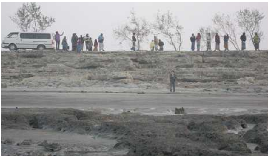
Fig. 4.11 Front side of the embankment in West Kuakata
