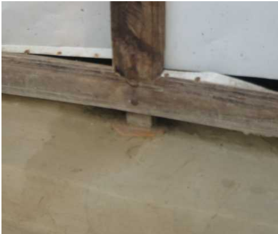
Fig. 4.14 Foundation of the fisherman's house
