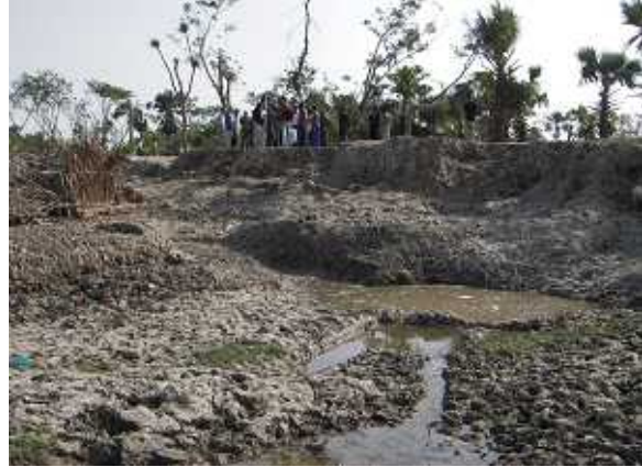
Fig. 1-3-5 Outer sea banks damaged by the storm surge
