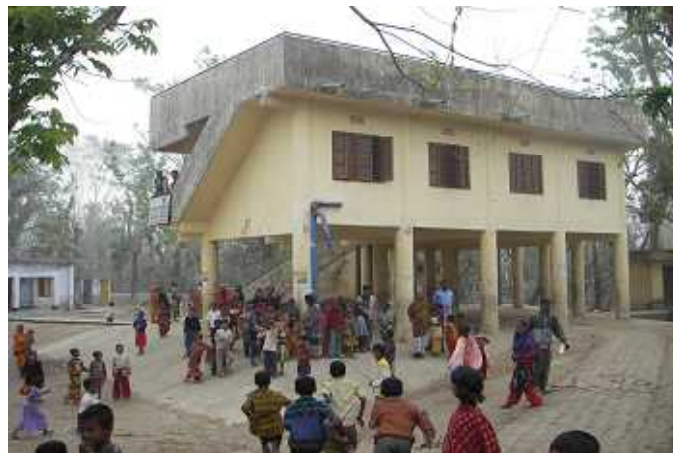
Fig. 1-2-1 A Cyclone Shelter, Kadamthala in Roenda Bazar
