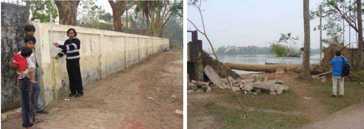
Fig. 1-3-1 Flood mark at BWDB local office at Pirojpur
