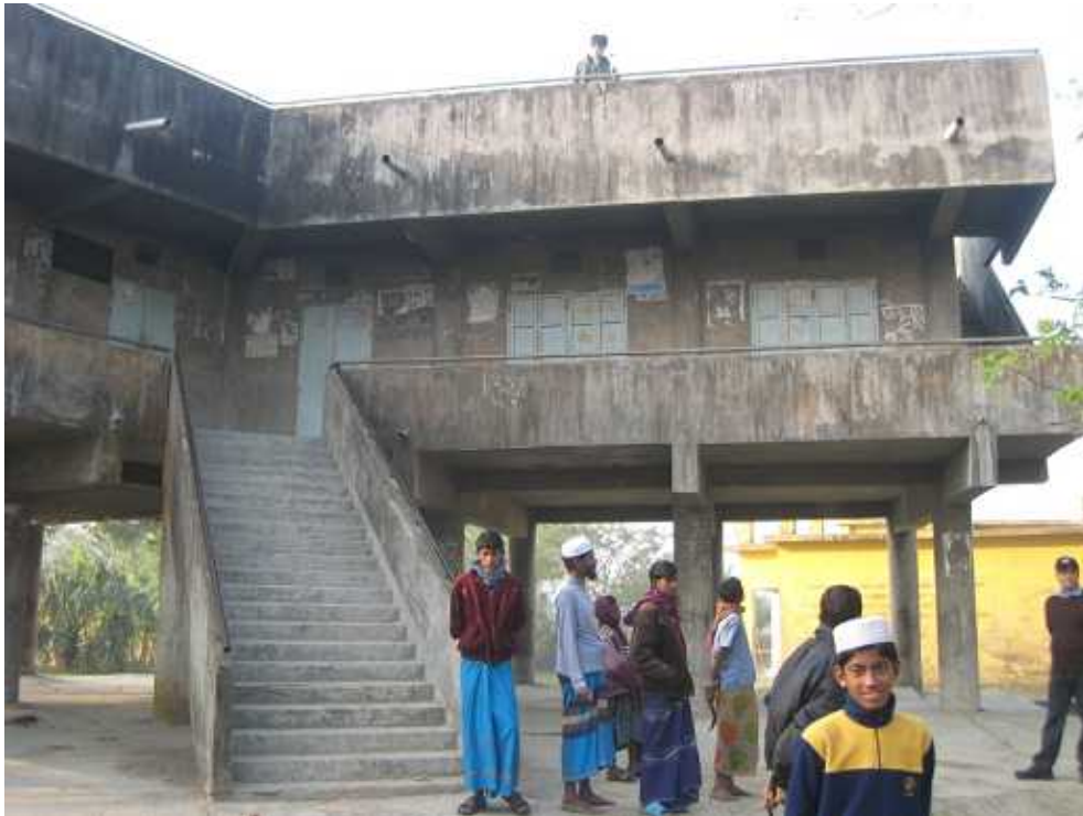
Fig. 4.5 The shelter in West Kuakata was built in the school where is about 610m away from the embankment. .
