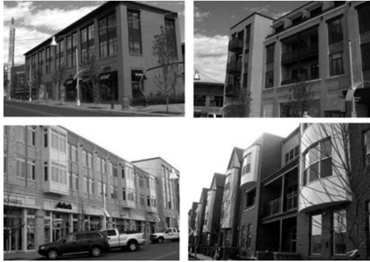
Belmar included a variety of housing types and architectural styles. Courtesy Continuum Partners LLC.
