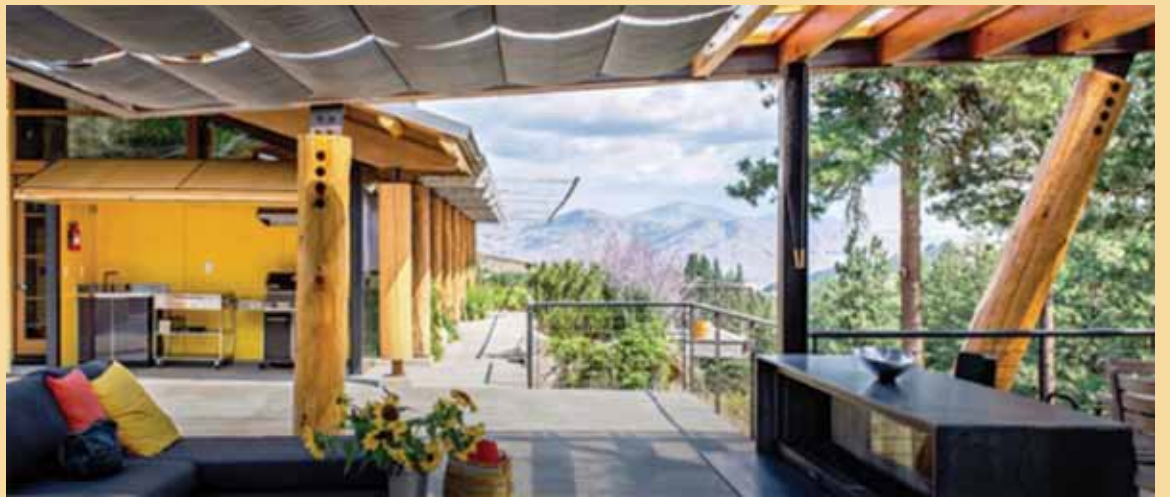
(An Elbow Coulee Remodel courtesy of PBW Architects will be featured in "Embracing the Outdoors" the 18th Annual Methow Valley Home Tour.)
