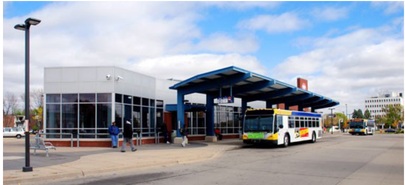
Figure 1: Brooklyn Center Transit Center
