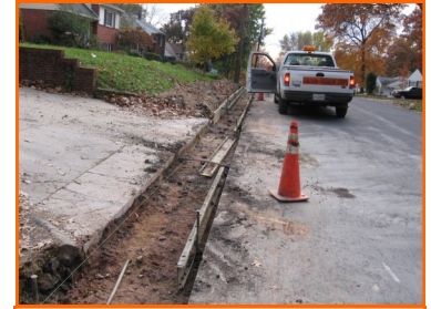
Curb forms being made ready for concrete
