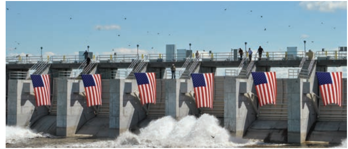
The all-new, improved Minidoka Dam and spillway reopened for business in May 2015.
