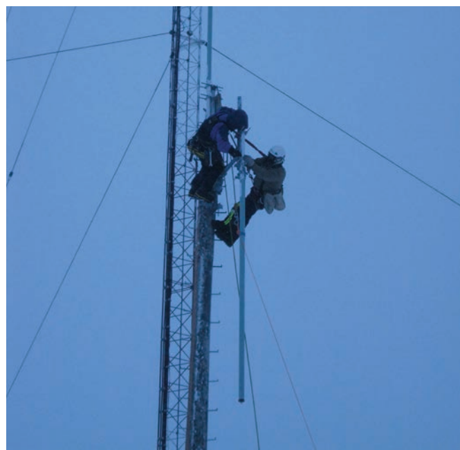
Cell tower technicians work in rugged conditions in northwest, Arctic Alaska.
