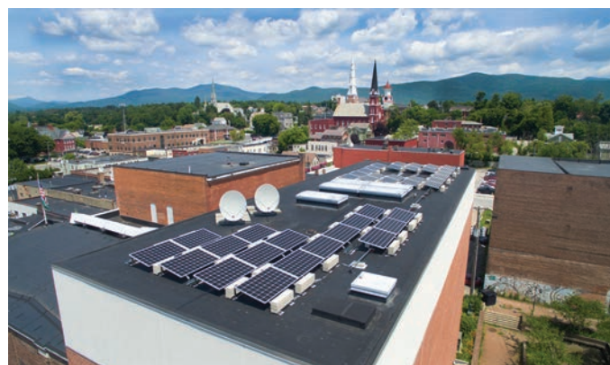
Solar panels on the roof of the Paramount Theater. The improvements have energized downtown Rutland, bringing more patrons to the Paramount and neighborhood small businesses.
