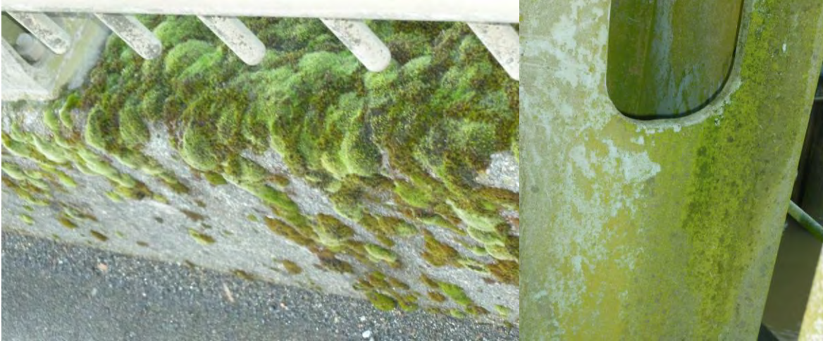
Figure 6. Hoquiam River Riverside 1417 Bridge
