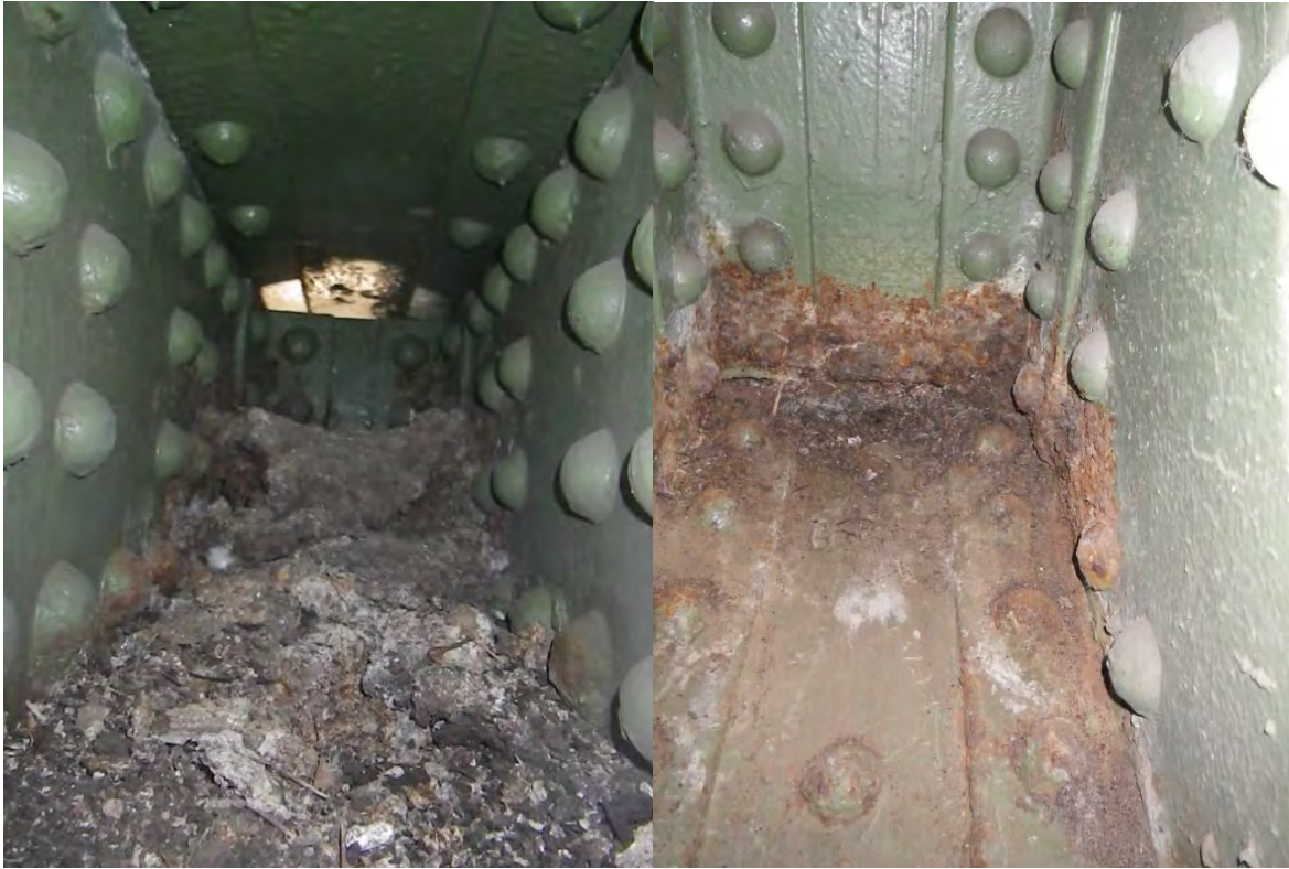
Figure 2. Bottom chord interiors
