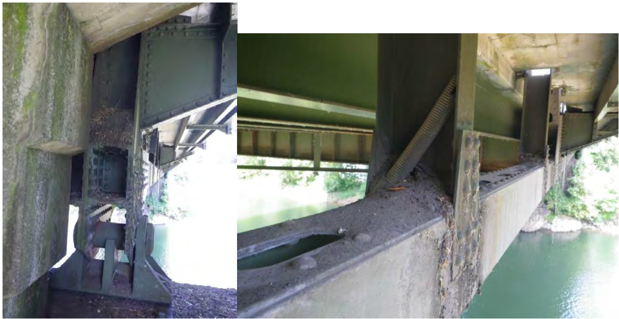
Figure 1. Bottom chord ends
