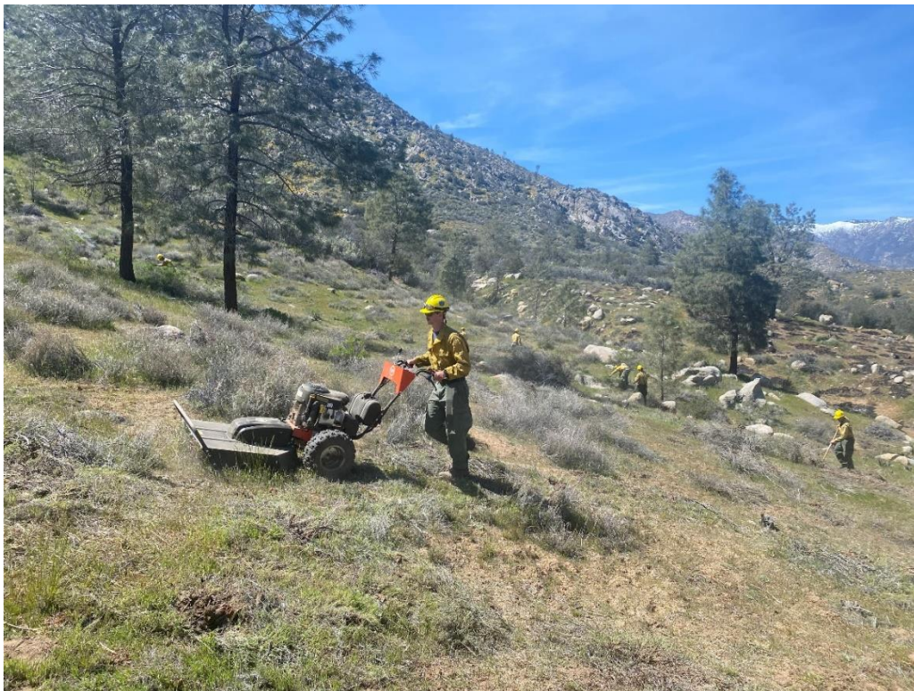
Fuels crew utilizing brush mower on hillside to remove sage along fuel break in Battalion 7.
