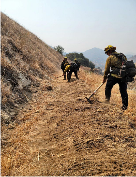
Figure 9 CAL FIRE hand crew constructing a fuel break.
