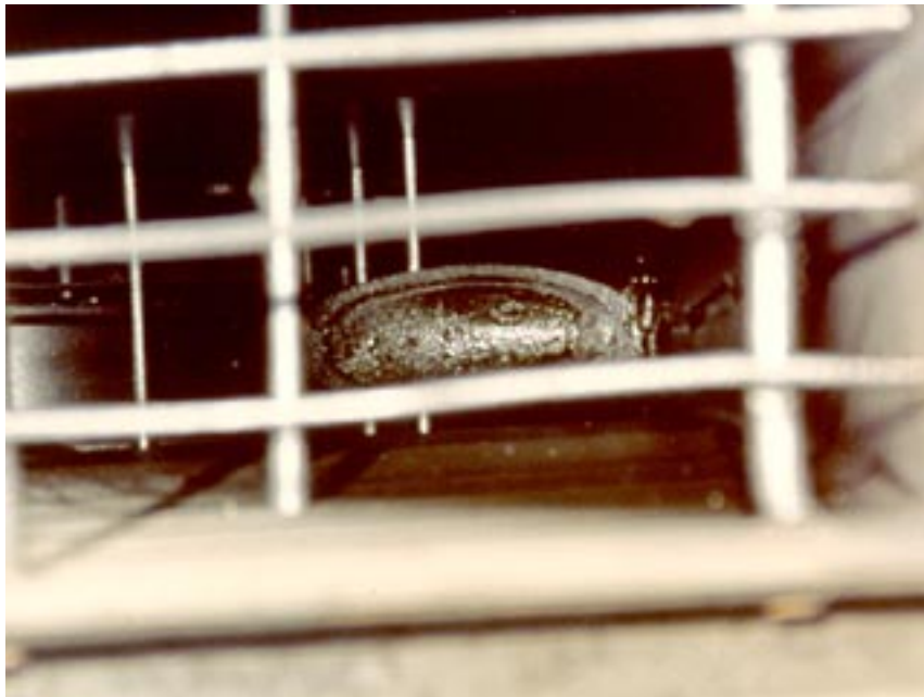
Photograph 5-14. Looking Down Exhaust Stack with Eductor Tube
