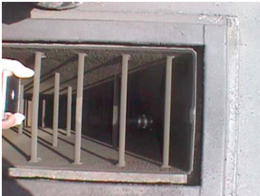
Photograph 5-16. Looking Down Exhaust Stack with Eductor Tube
