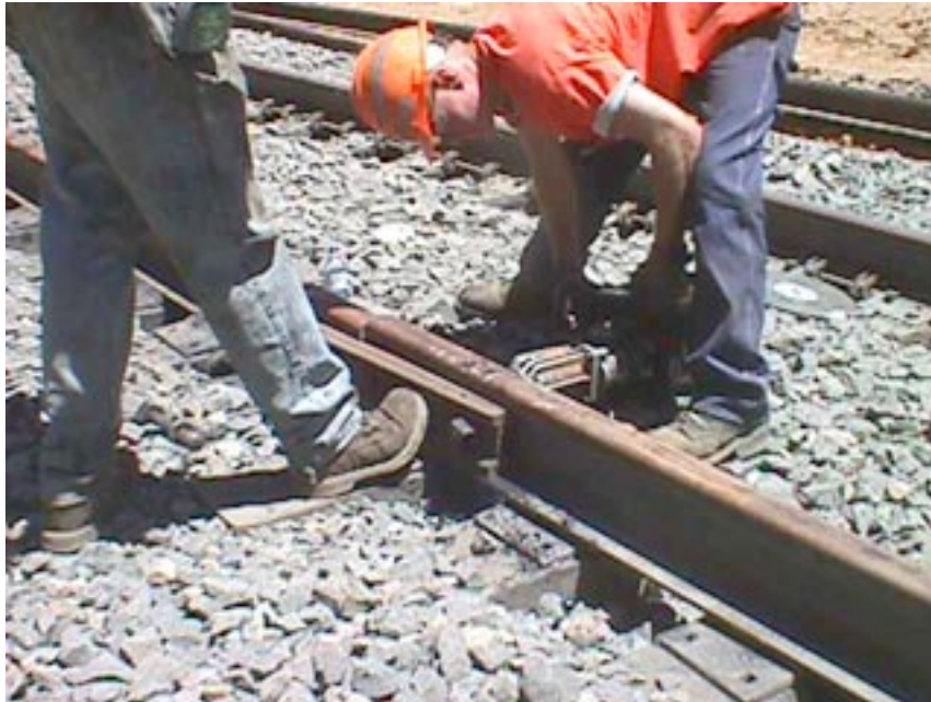
Photograph 7-12. Gas-Powered Impact Wrench in Use
