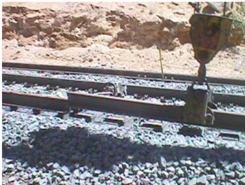
Photograph 7-5. Replacing Rail with Pettibone Crane
