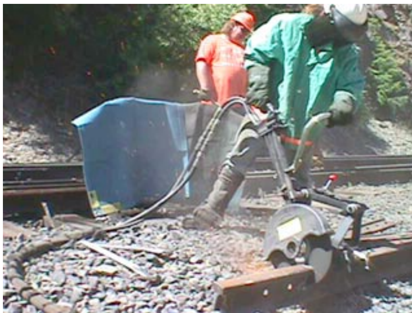
Photograph 7-16. Cutting Rail (Note Spark Guard and Backpump)
