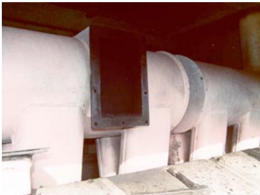
Photograph 5-6. Exhaust Clean-Out Trap on Non-Turbo Engine
