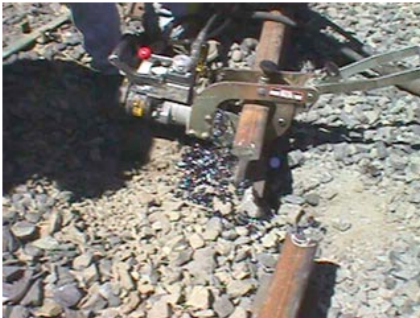
Photograph 7-19. Pneumatic Drill with Hot Shavings
