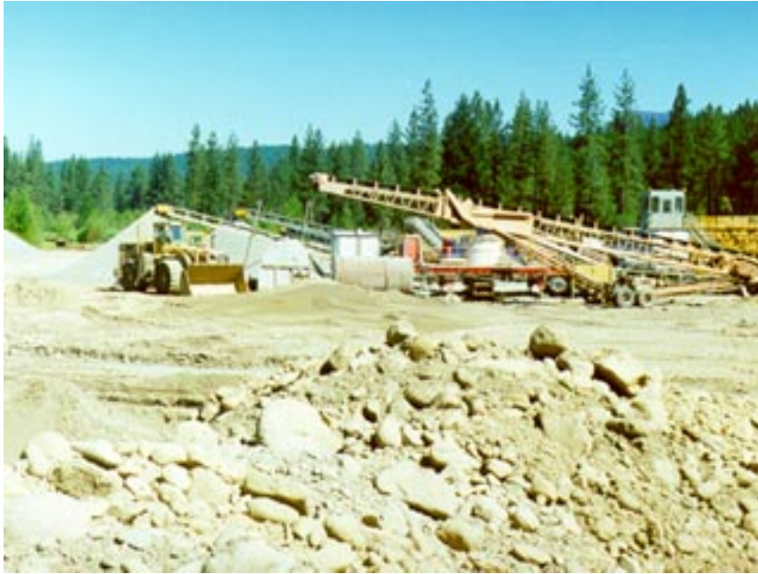
Photograph 10-6. Rock Crushing Operation
