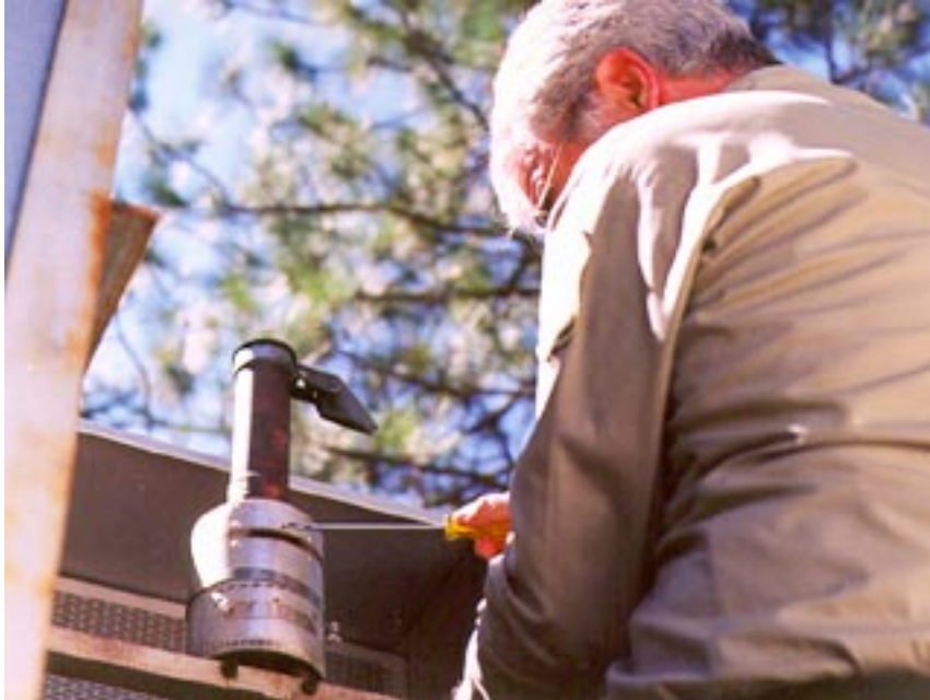
Photograph 9-6. Spark Arrester with Band Removed
