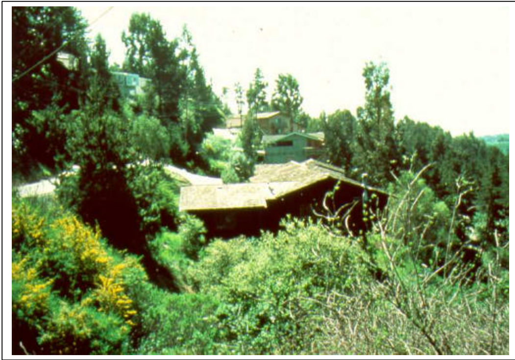
Photograph 4.2. Special Fire Problems in Rural Areas
