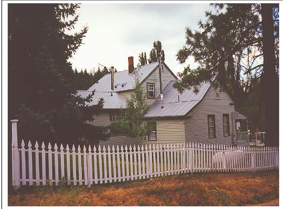
Photograph 9.4. Class A Roof
