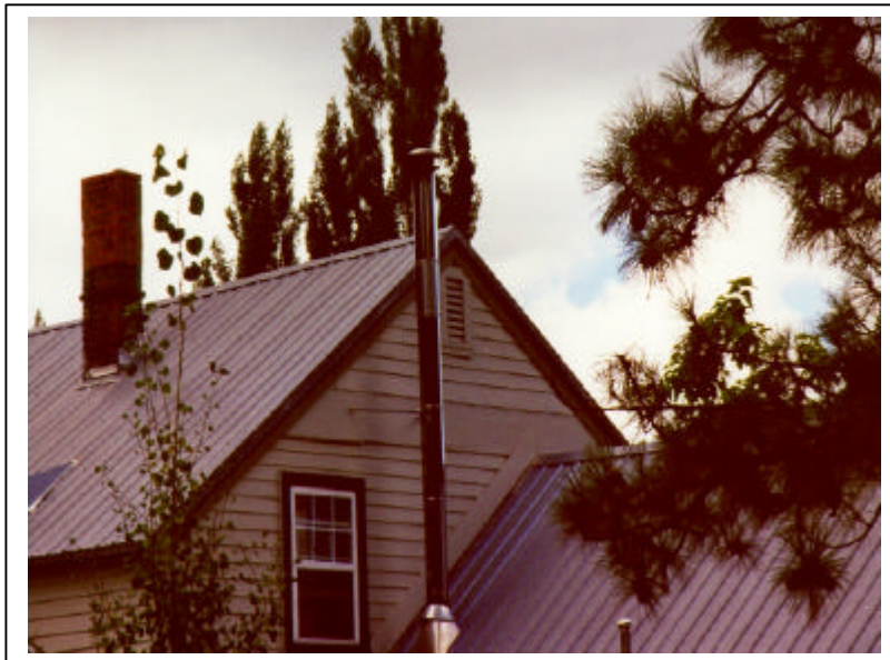
Photograph 9.5. Dormer Vent and Chimneys
