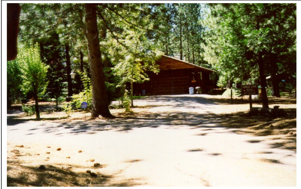
Photograph 8.2. Roadway to Rural Structure
