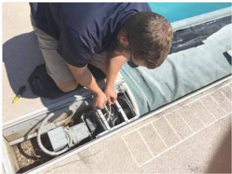
As part of the inspection process, technicians need to ensure proper tension on the rope reel tension blocks.
