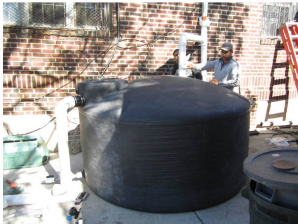
Neighborhood Center cistern
