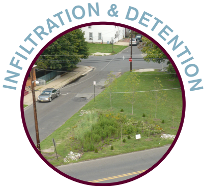
Ferry Avenue Rain Garden: This demonstration project was designed on a vacant lot owned by CCMUA to intercept runoff from surrounding roadways. The completed 900 square foot rain garden can capture, treat, and infiltrate over 75,000 gallons of stormwater each year. | Photo courtesy of CCMUA
